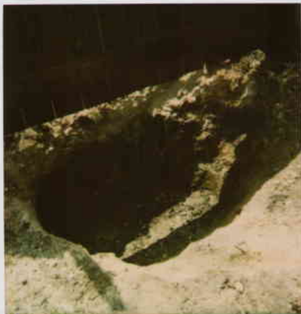
5/20/97 Contaminated soil (OE) excavated from pile.
