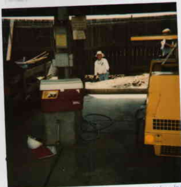
Contaminated soil behind carport/car wash area. 5/20/97
