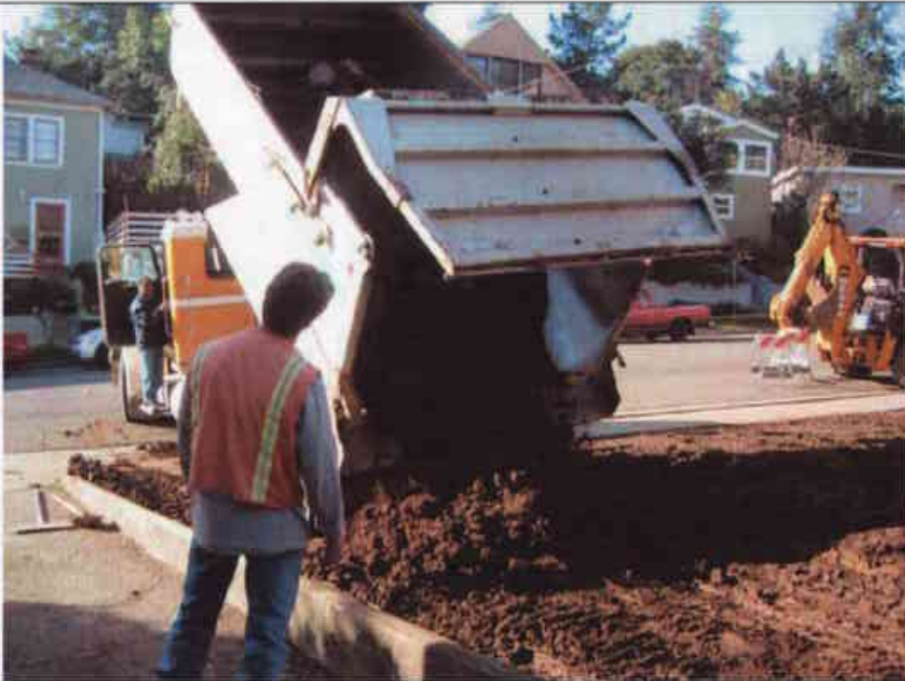
Importation of backfill materials.
