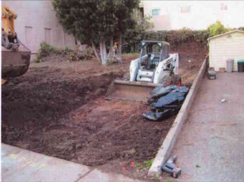
Completion of excavation to two feet below ground surface.
