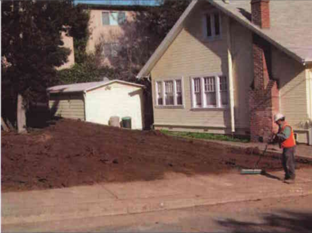
Completion of backfill and compaction activities.
