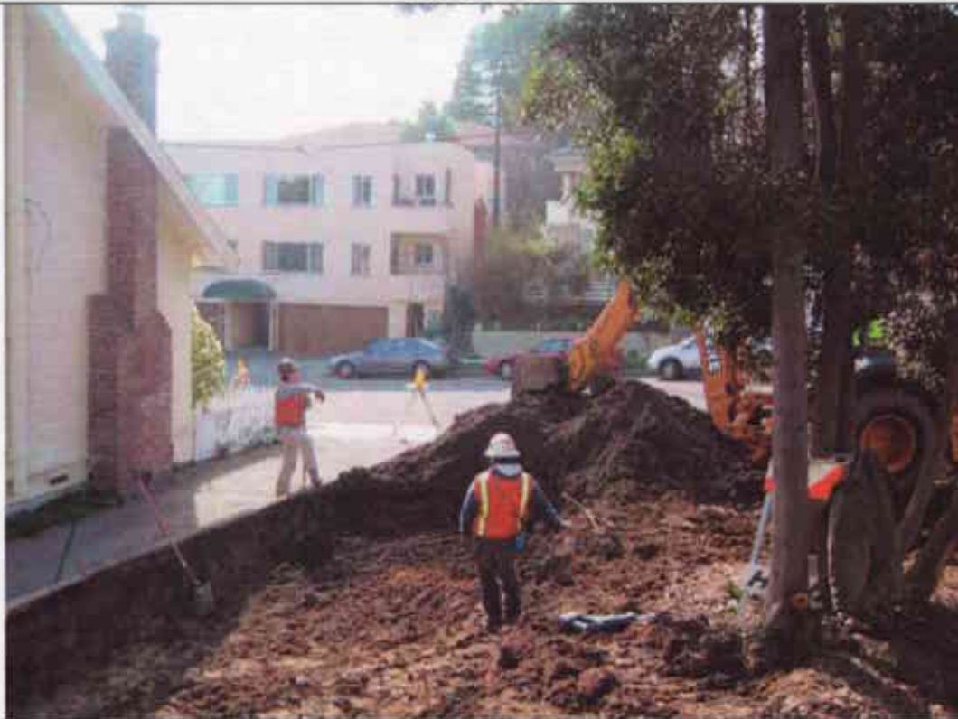
Excavation of impacted soils, south end of site.
