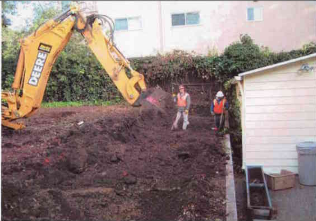
Excavation of impacted soils, north end of site.
