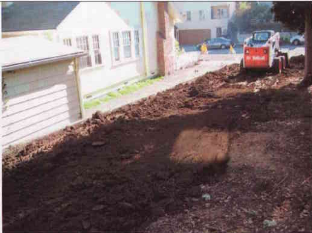
Emplacement and compaction of backfill materials.
