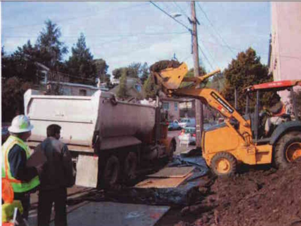
Loading and offhauling of impacted soils.
