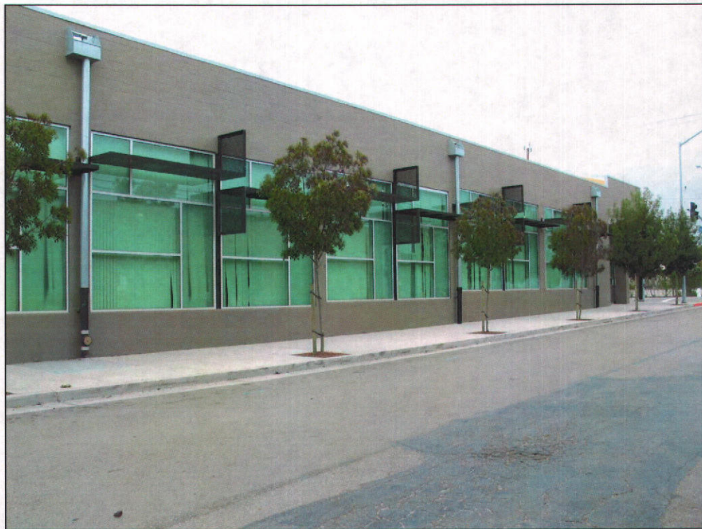
Photo 14 (Left-most leader in photo repaired)
