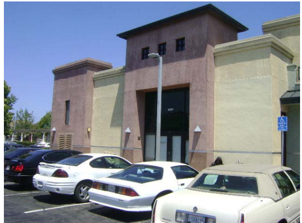
4. View of the west side of the smaller building.
