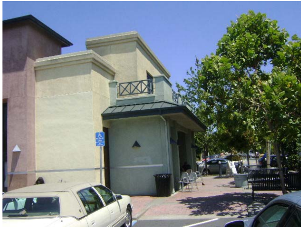
3. View of the south side of the smaller building.
