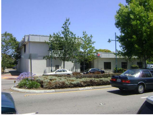
21. View of another adjacent property east (Bank of America).
