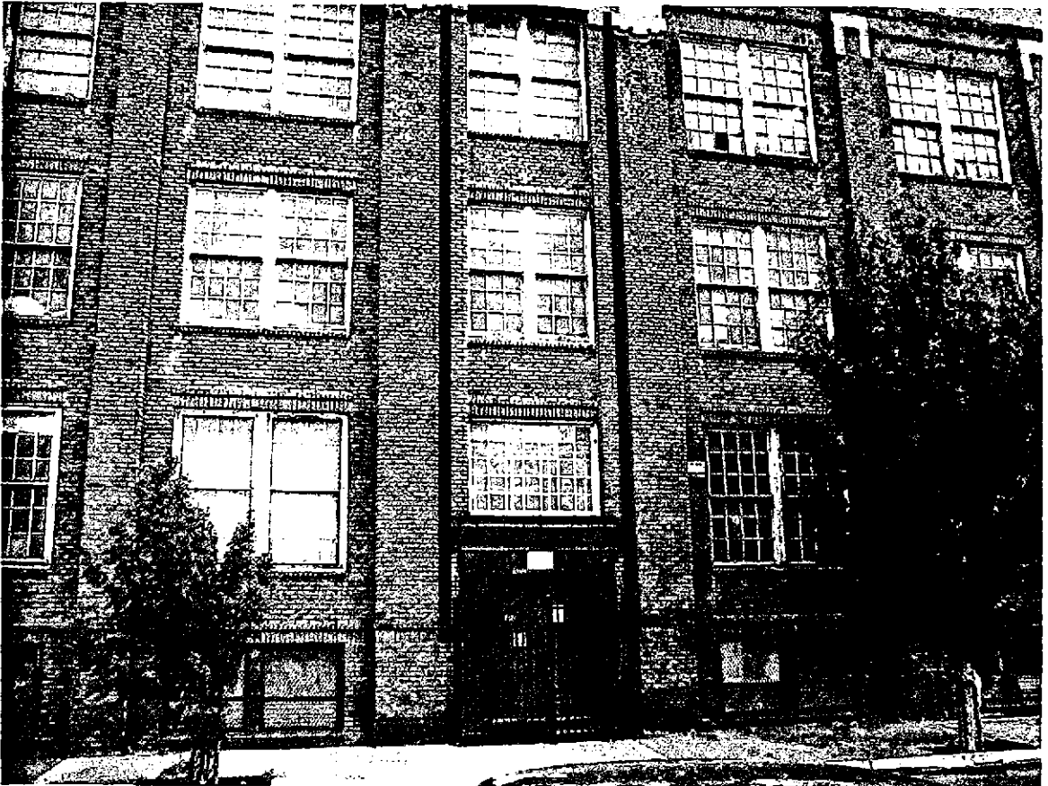
Photograph 2 – View to the Campbell Street side of the building.
