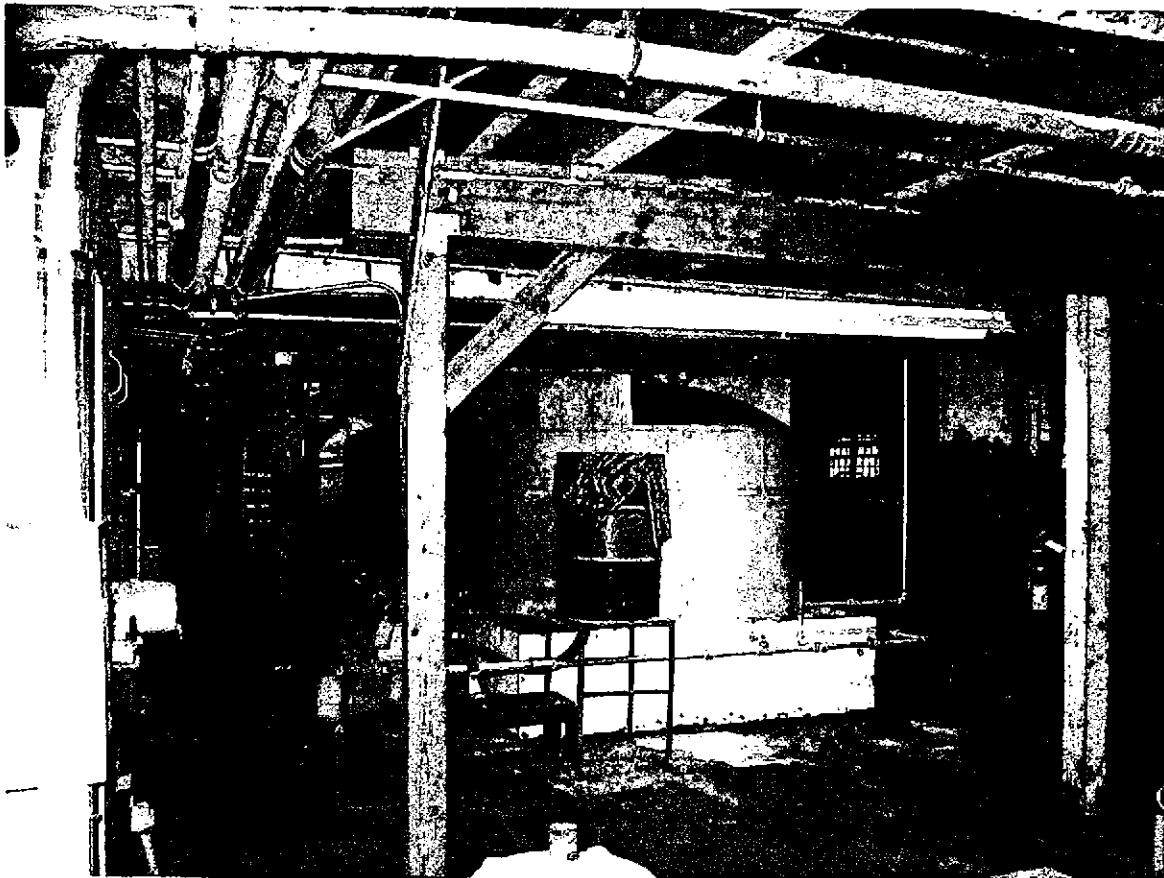
Photograph 4 – View of the latex mixing tanks in the basement.
