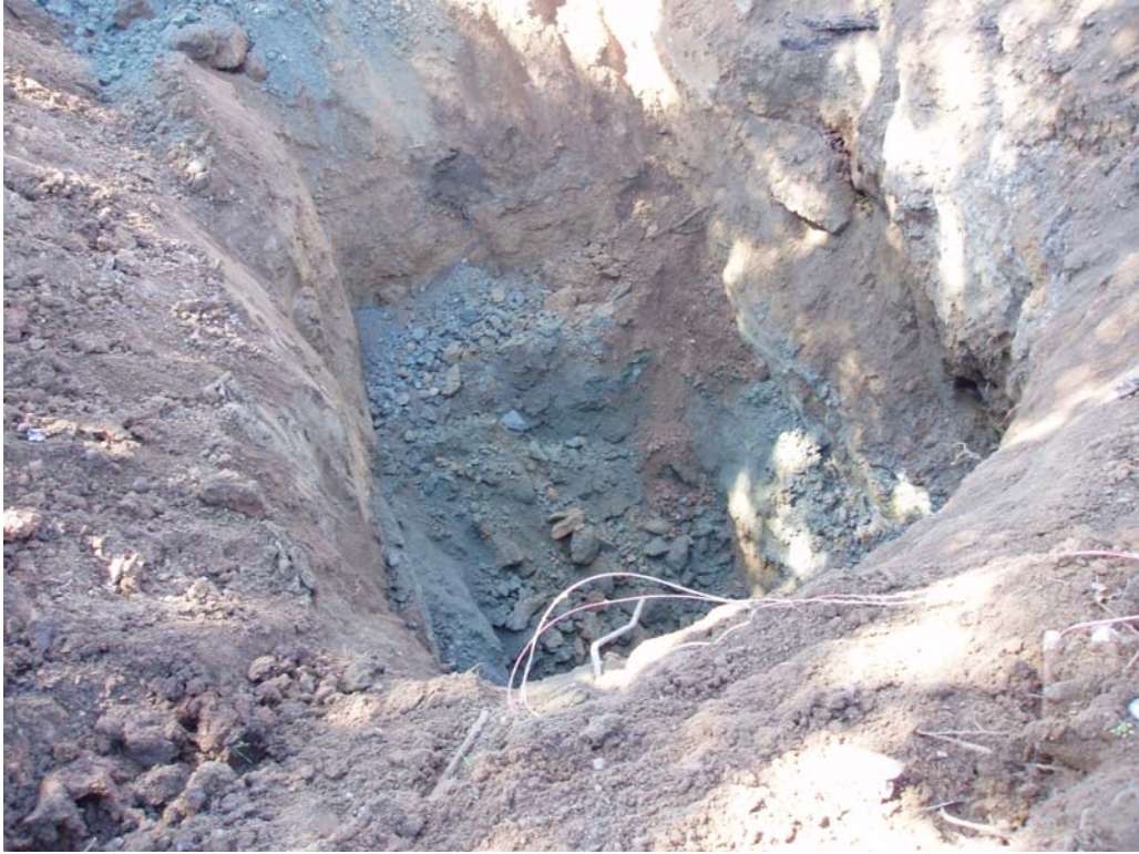
Photograph #5: Visible staining in soil around tank area.
