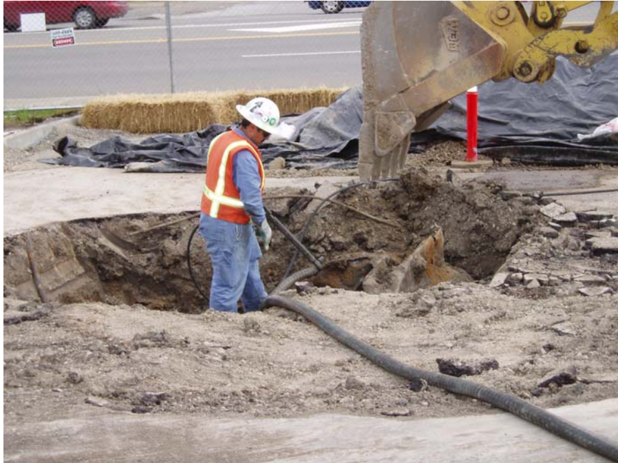
Photograph #1: Tank being cleaned.
