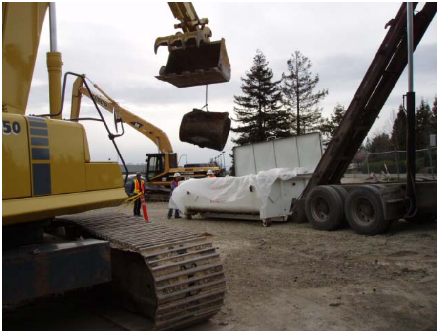
Photograph #4: Tank being loaded into the waste bin for disposal offsite.
