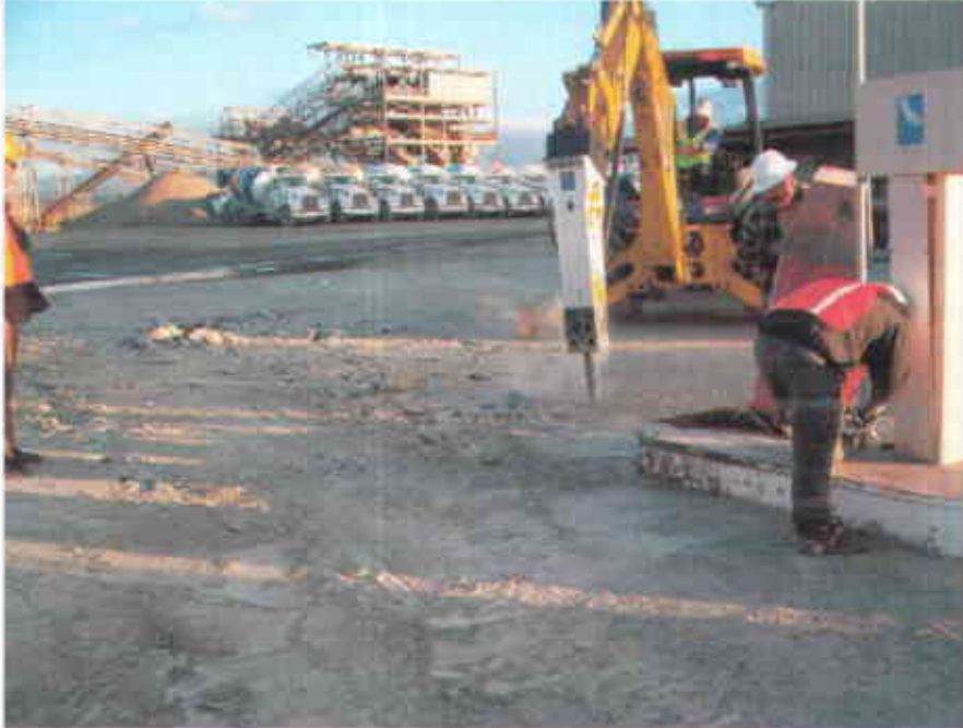
Breaking Concrete over Diesel Tank
