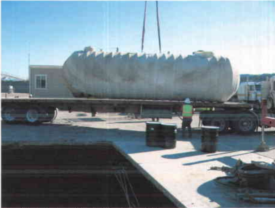
Gasoline Tank on Truck, Good Condition
