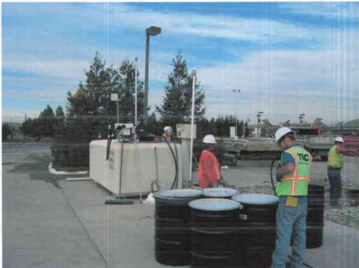
Pumping Gasoline to Above Ground Tank
