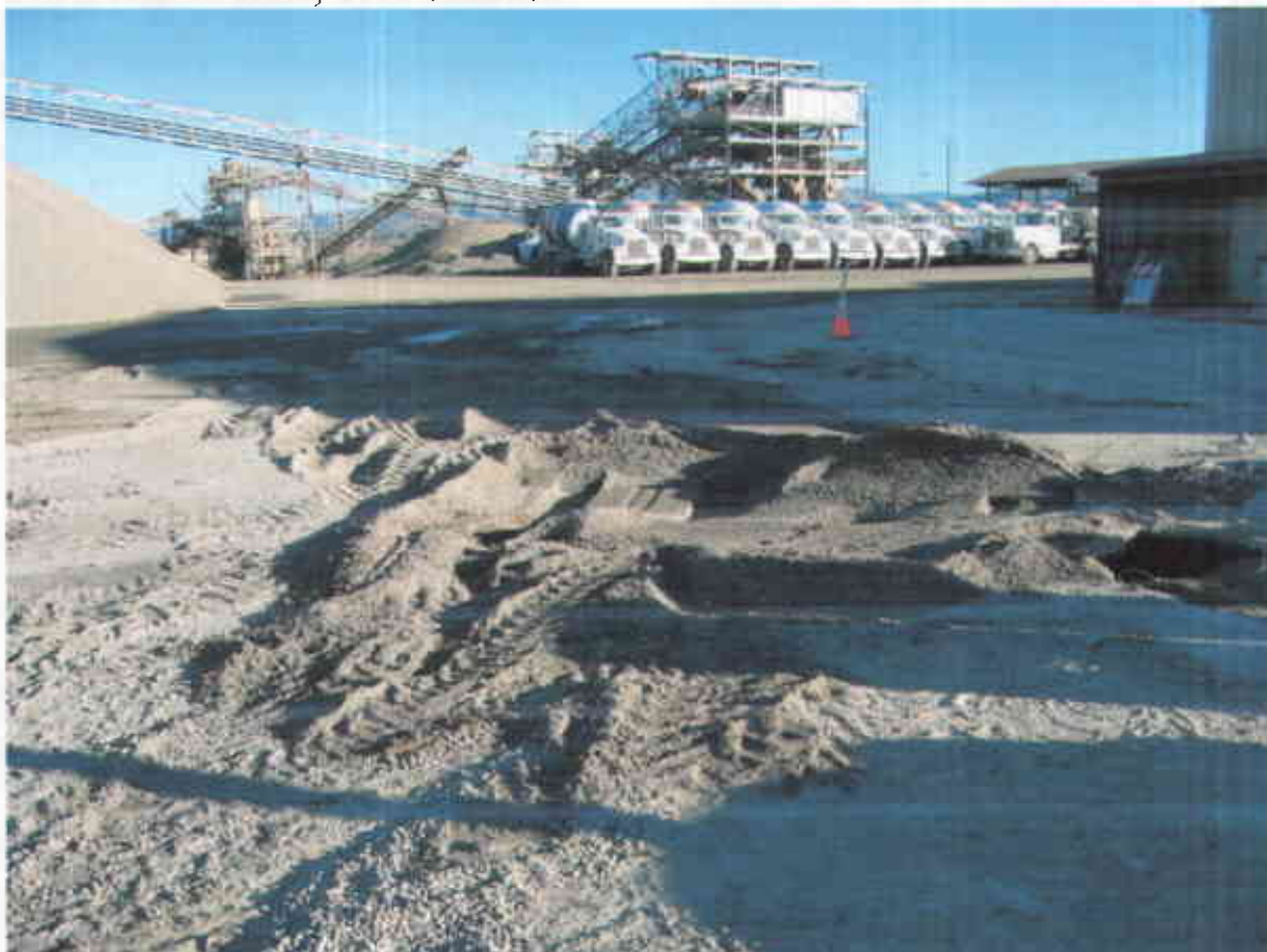
After Backfill, Diesel Tank
