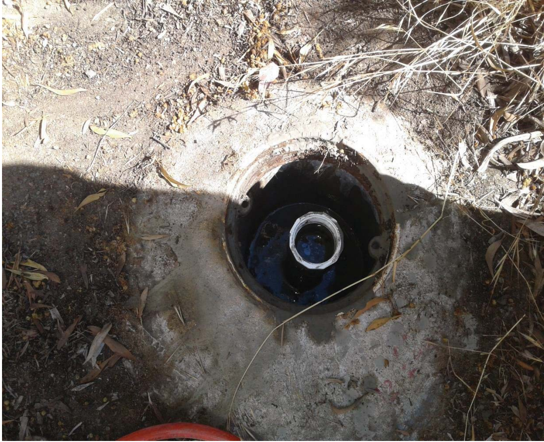
Abandonment of MW3
