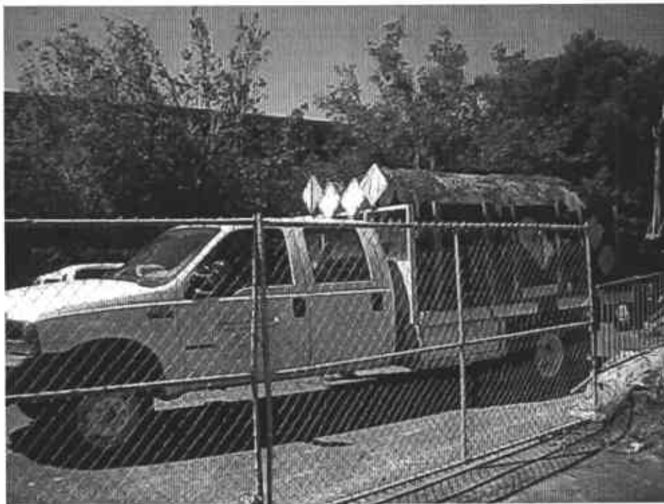
Tank Loaded on Truck; Ready for Disposal
