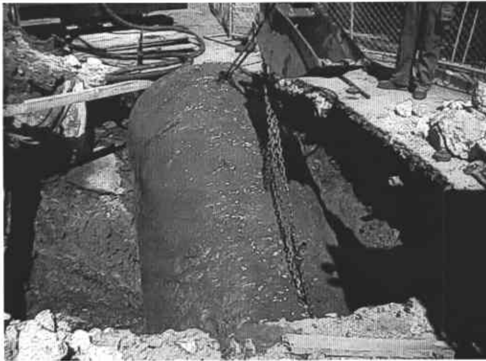
Tank in Excavation; Ready for Removal
