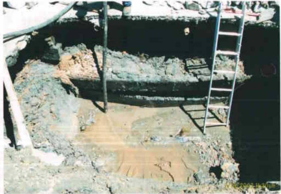
PUMPING CONTAMINATED H 2 O FROM EXCAVATION
