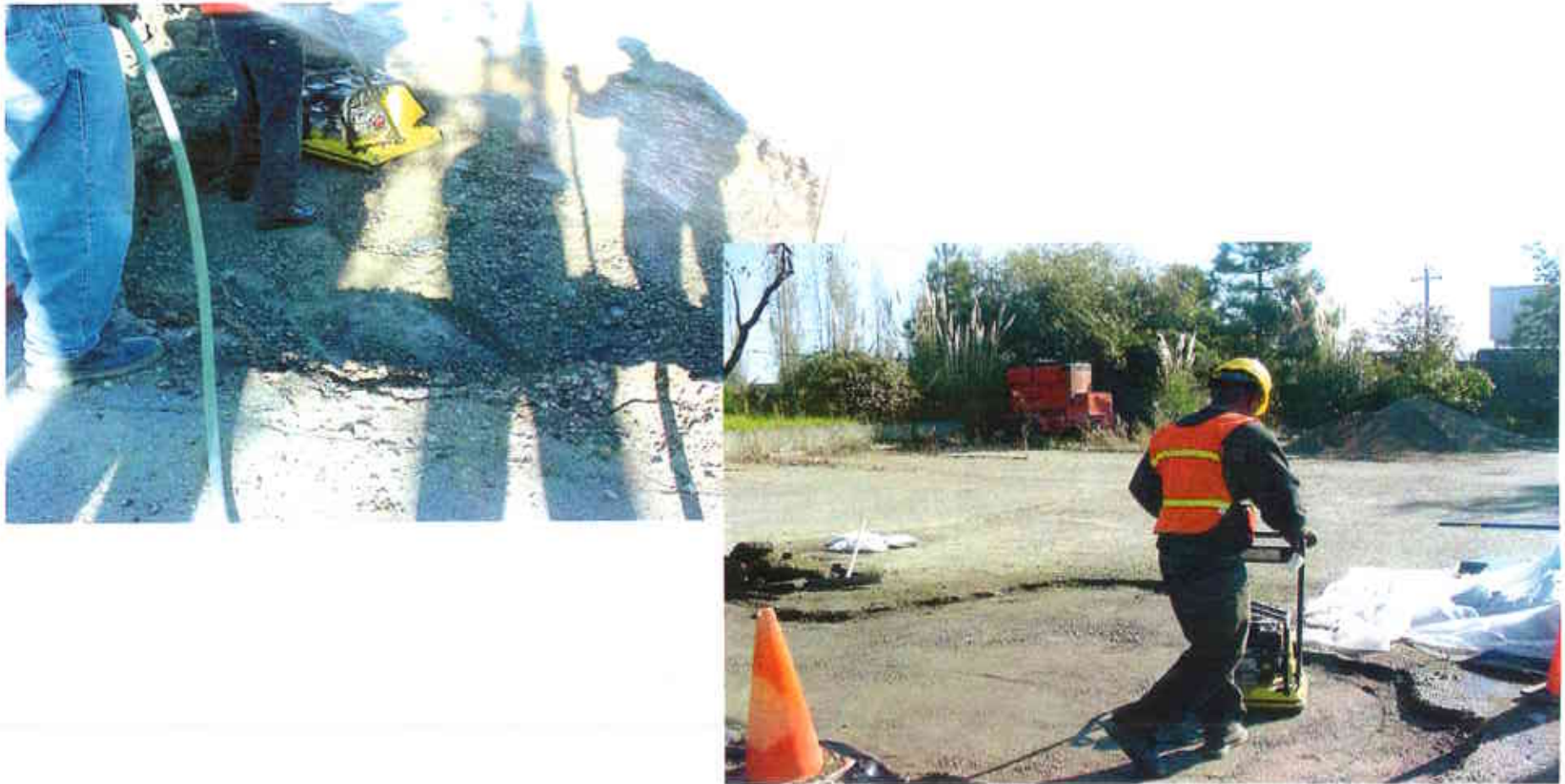
22. Use of vibratory-plate compactor on the emplaced backfill material
