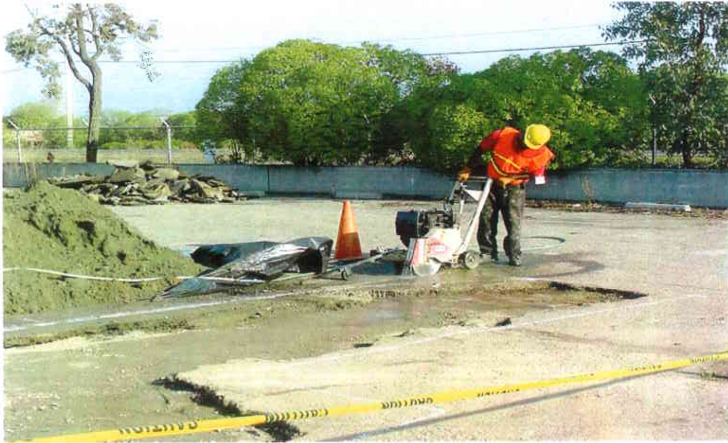
23. Saw-cutting to produce smooth pavement edges prior to paving
