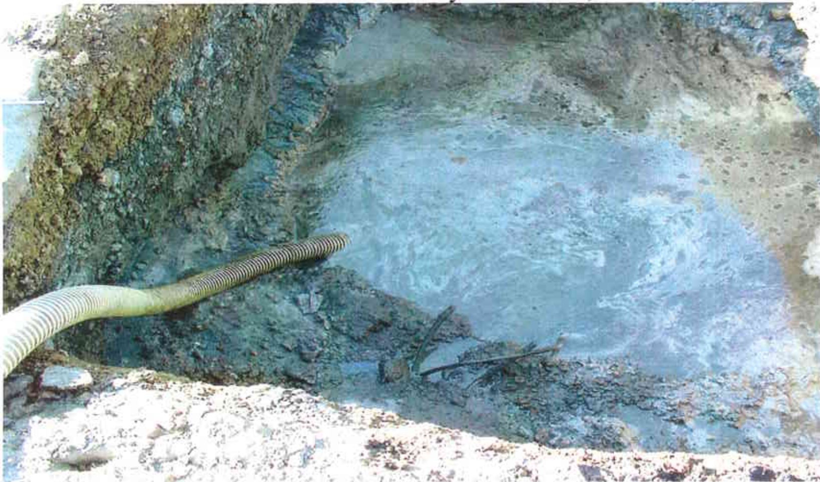
16. Excavation dewatering
