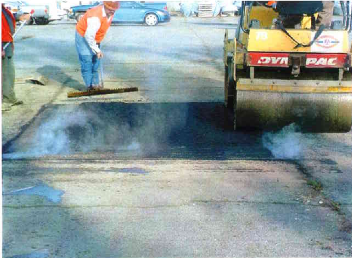
44. Compaction of hot asphalt with a wet roller
