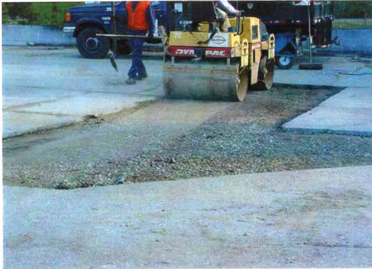
40. Final compaction with a roller prior to asphalt paving
