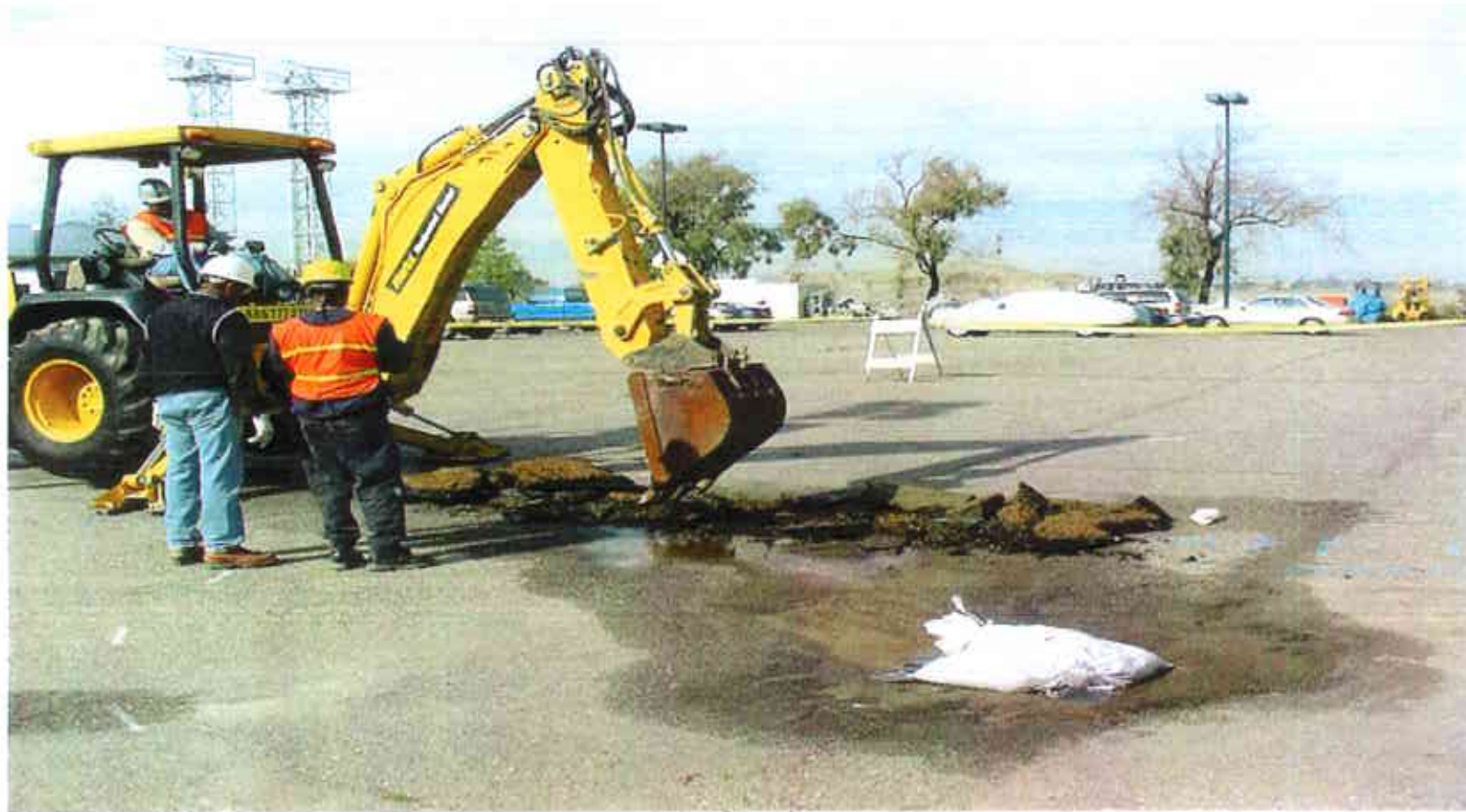
4. Use of Backhoe to breakup and remove pavement
