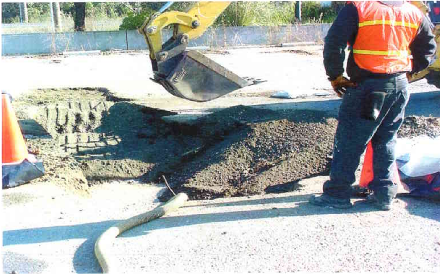
19. Backfilling of excavation (while excavation dewatering is continued)
