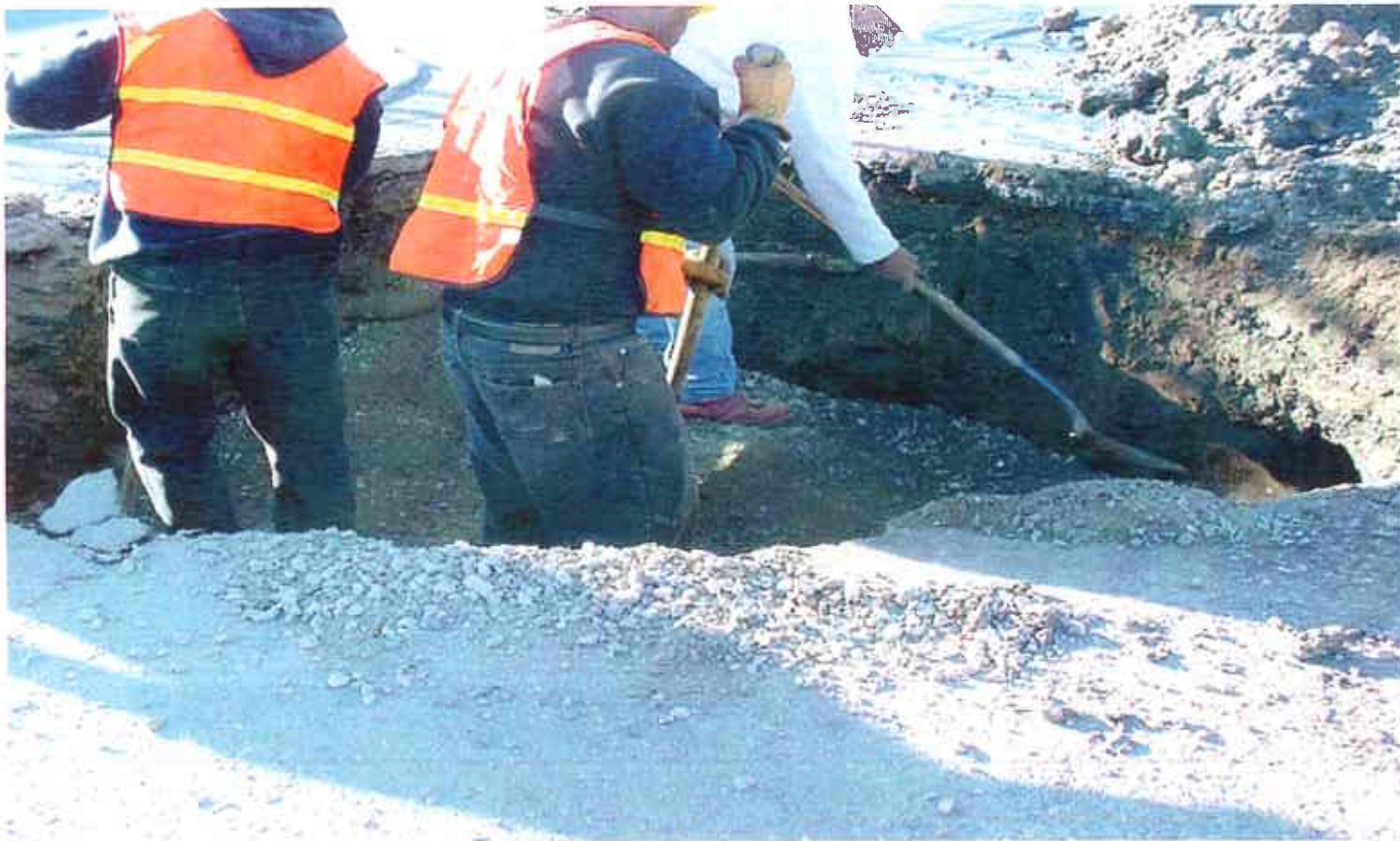
20. Manual spreading of the backfill material prior to compaction
