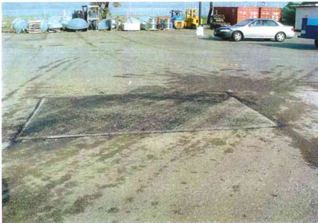
47. Resurfaced area at the former location of UST No. 6
