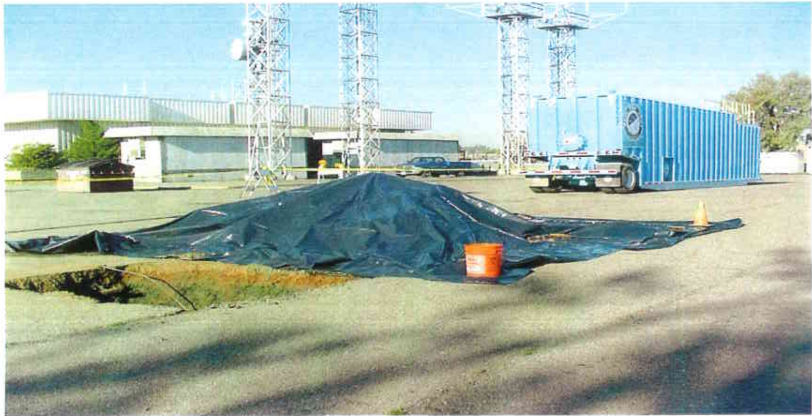
17. Covering of soil stockpiles with Visqueen
