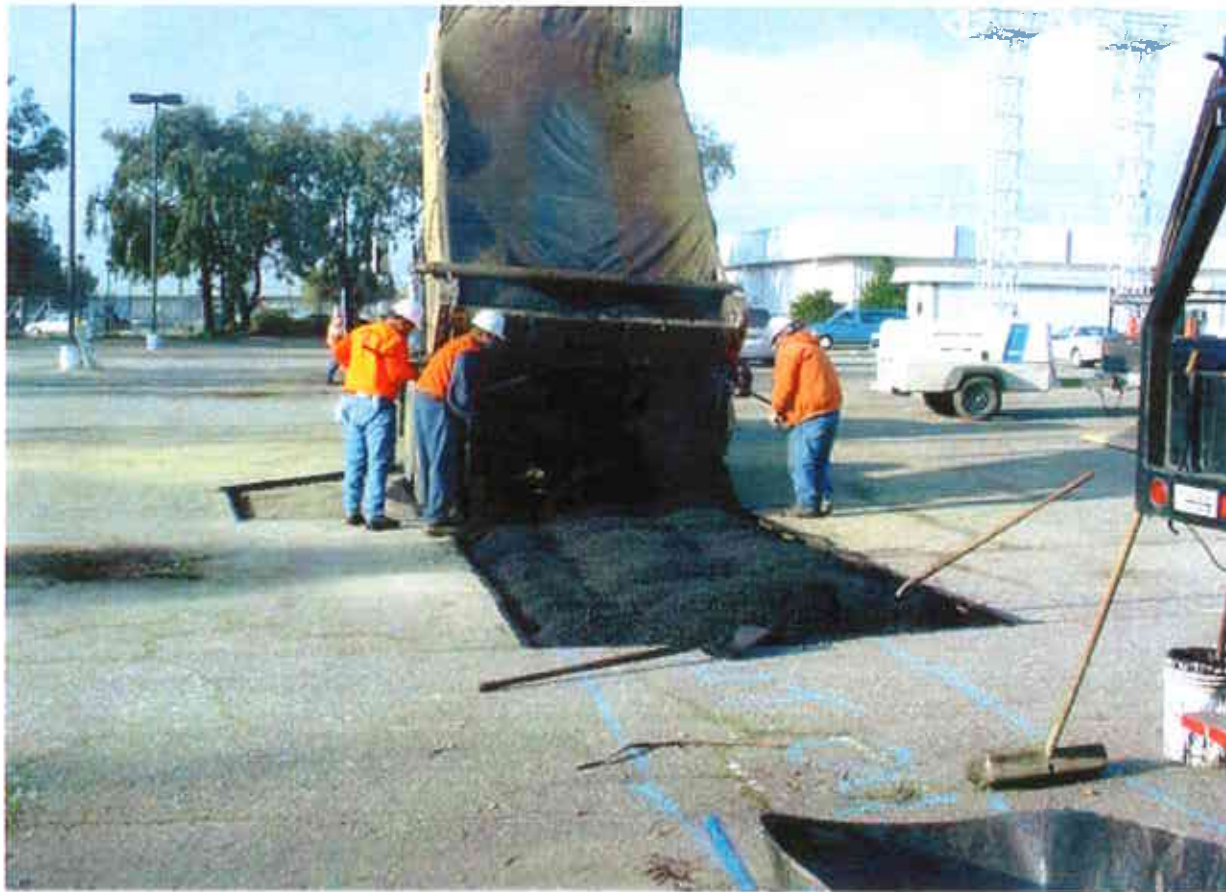
42. Placement of fresh asphalt onto the surface of the compacted area
