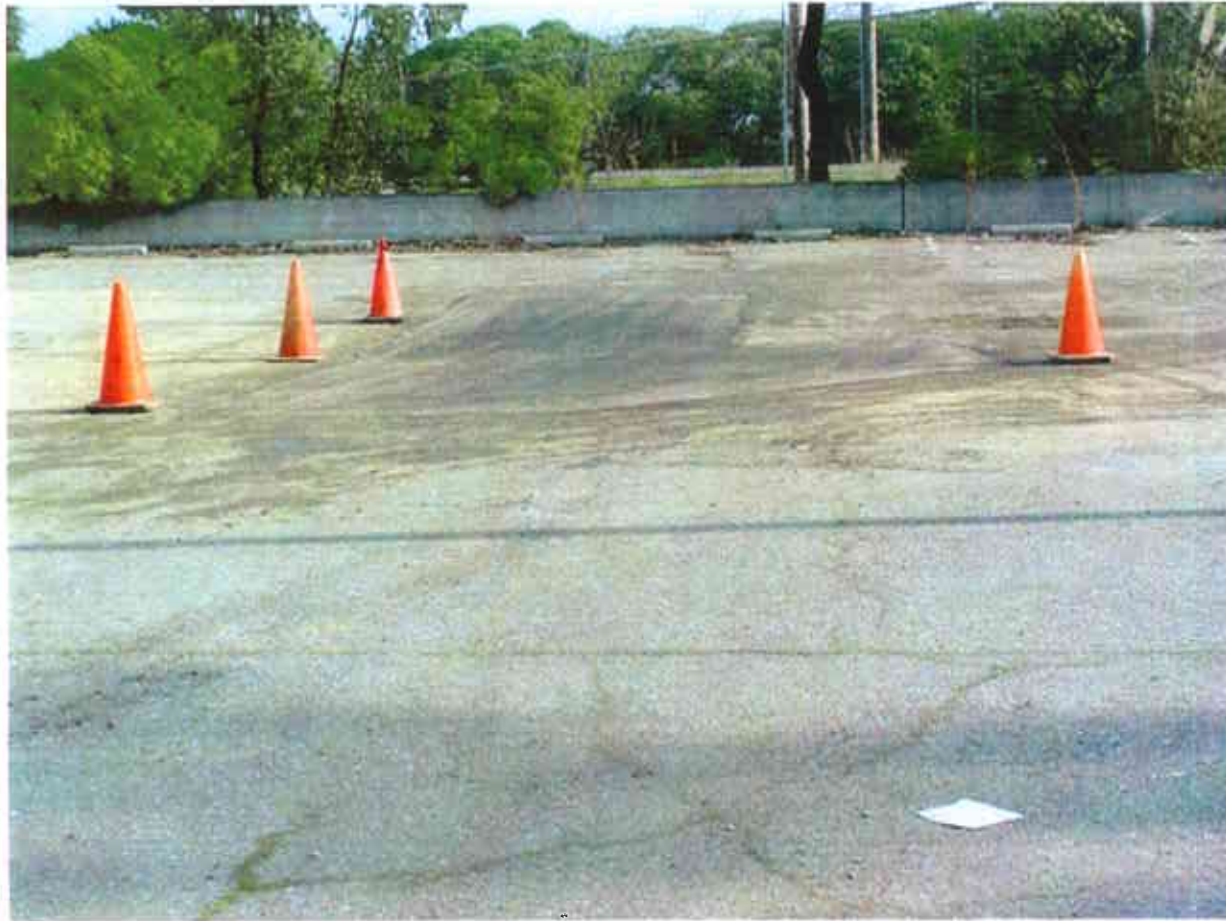
45. Resurfaced area at the former location of UST No. 8
