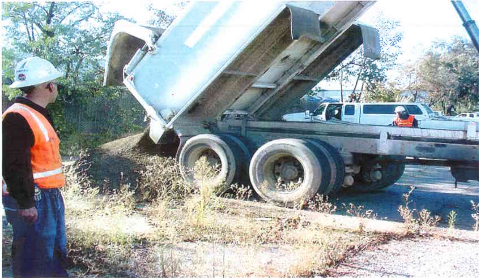
18. Imported clean backfill material being delivered to site
