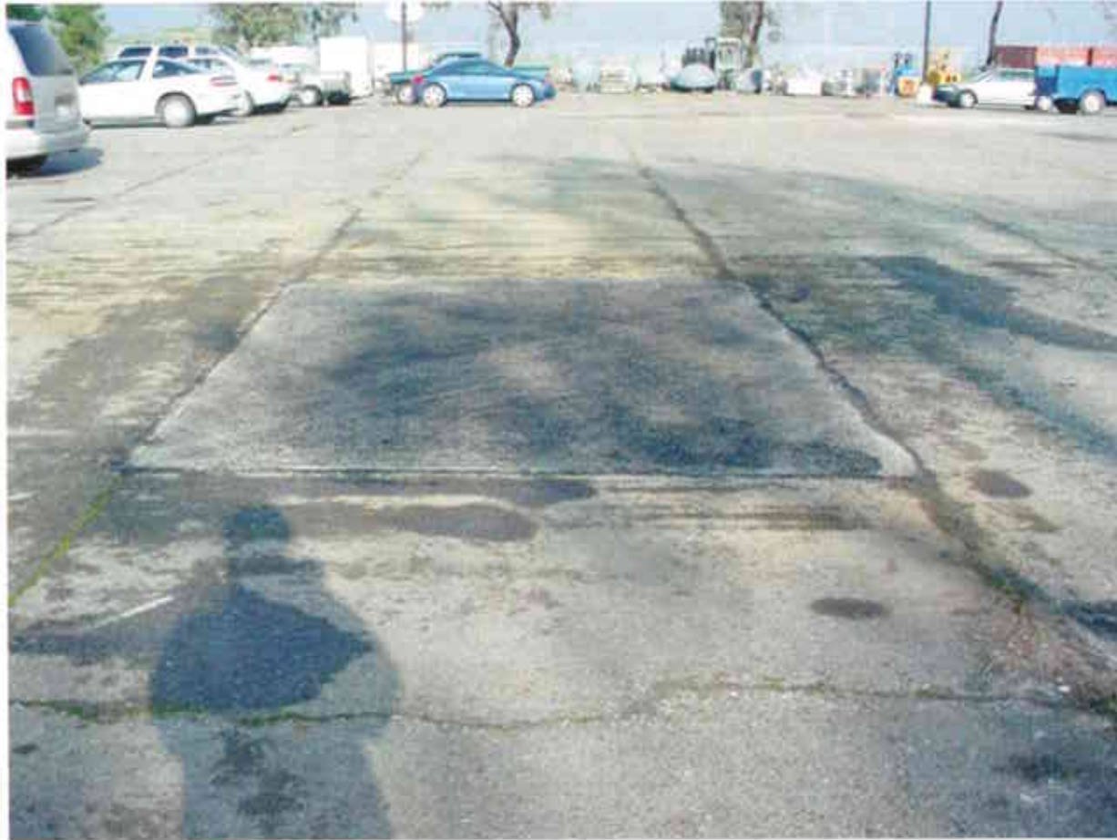
46. Resurfaced area at the former location of UST No. 7
