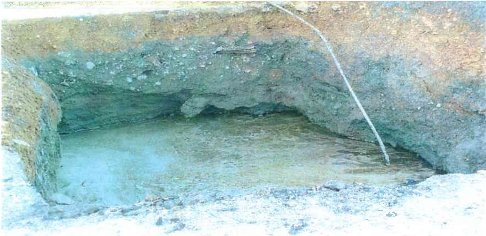
14. Water accumulation in the excavation for UST No. 6
