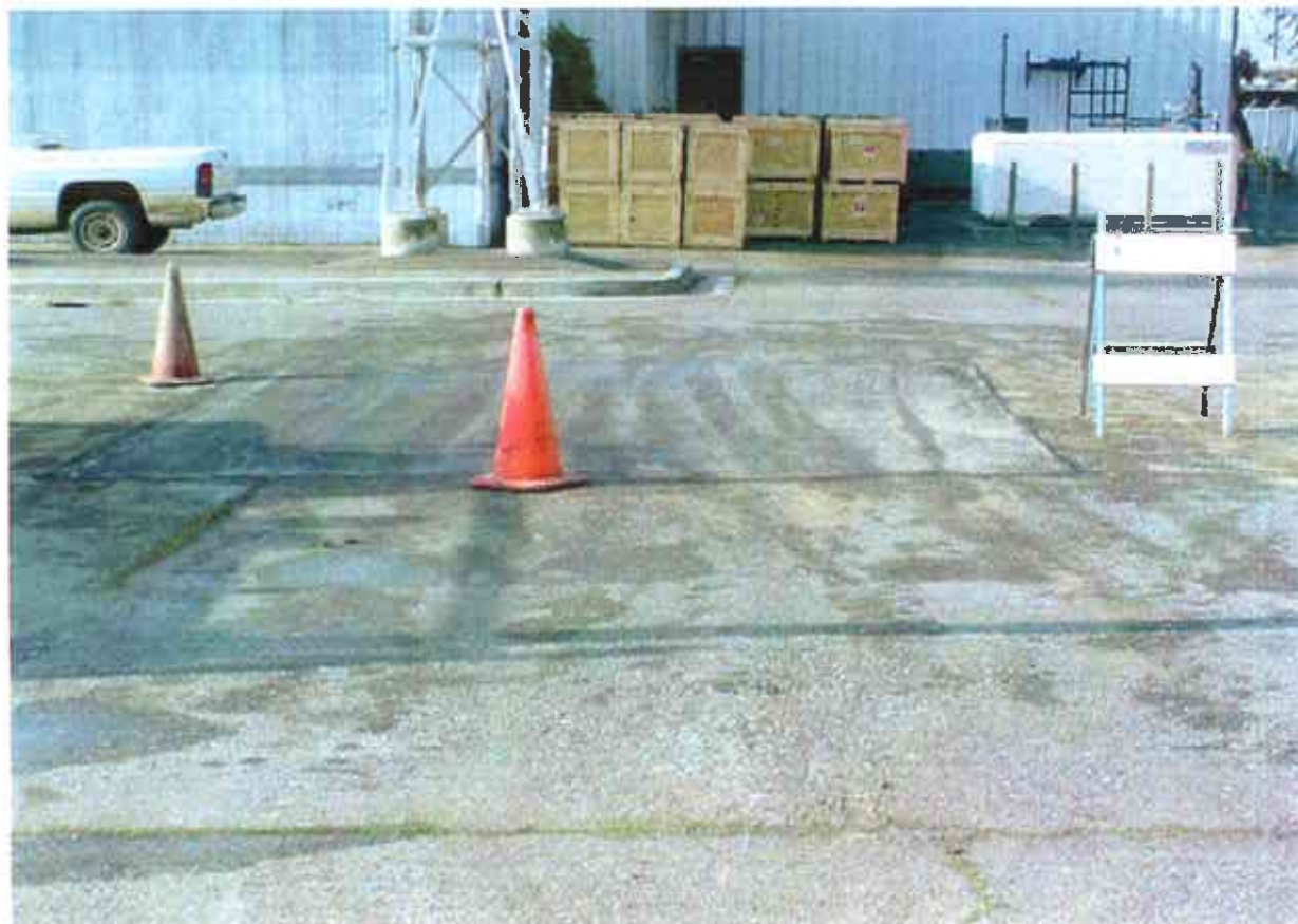
48. Resurfaced area at the former location of UST No. 5
