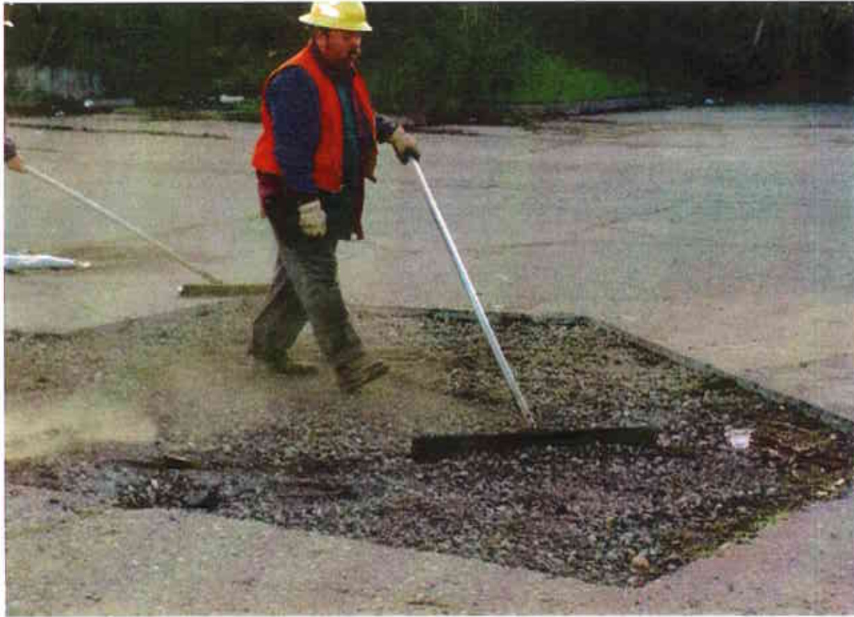
38. Smoothing the base prior to further compaction and asphalt paving
