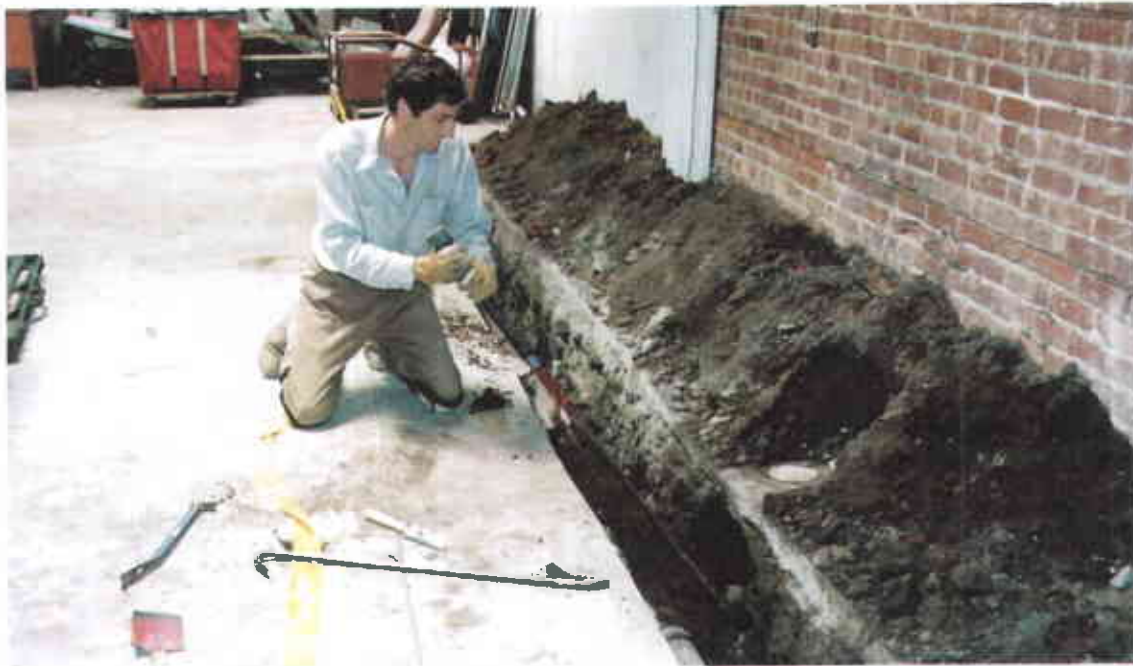
Subject: Hand auger sampling beneath sanitary sewer line floor drain
