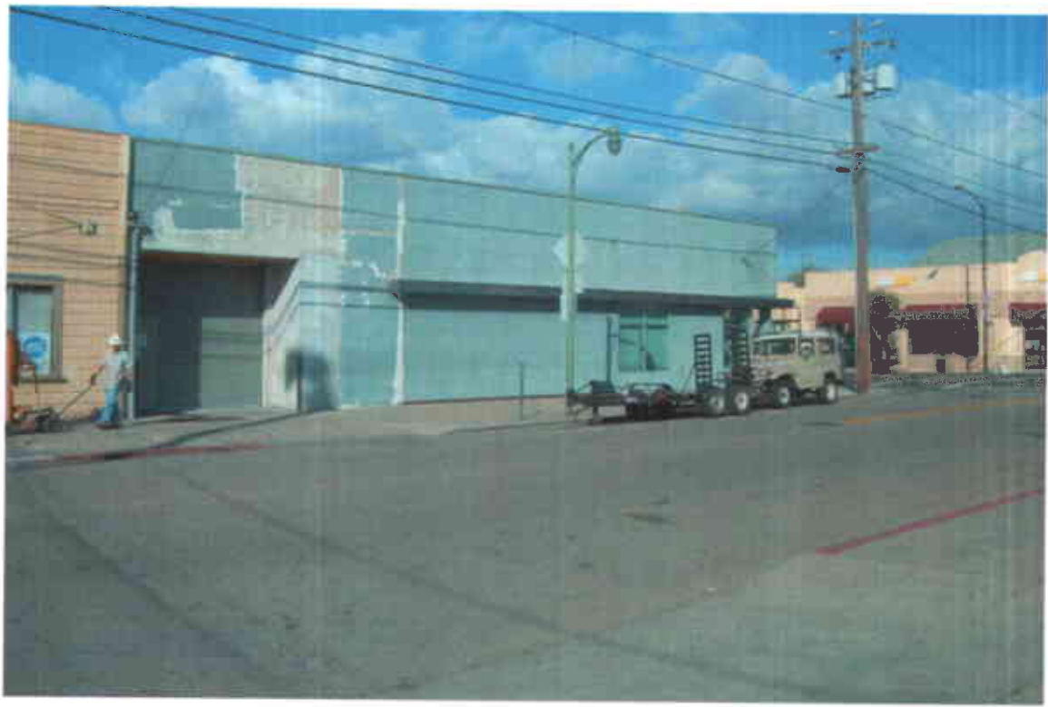
Photograph 3 – View to the northeast of 1701 Webster St. from across Pacific Ave.
