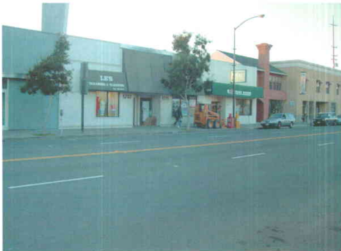
Photograph 2 – View to the northwest of 1701-13 Webster St.
