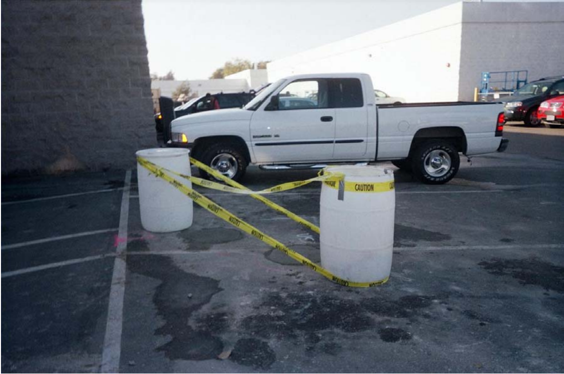
Photo 16: SB-9 and VAS-1 concrete completion.
