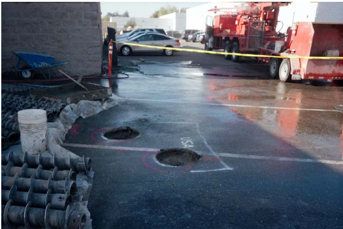
Photo 9: SB-VAS-1and SB-9 post drilling, pre concrete.
