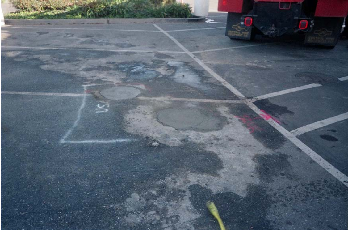
Photo 12: SB-9 and SB-VAS-1 Concrete Completion
