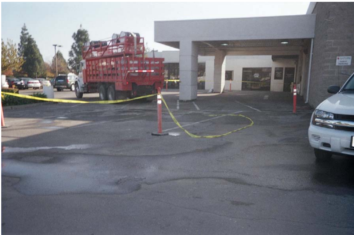
Photo 13: Work Area post drilling activities.
