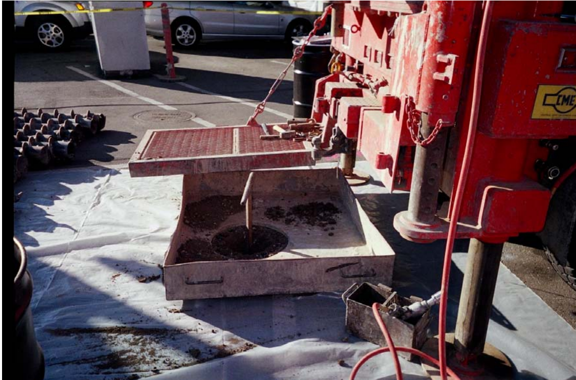
Photo 1: Hand auger to 5 ft bgs
