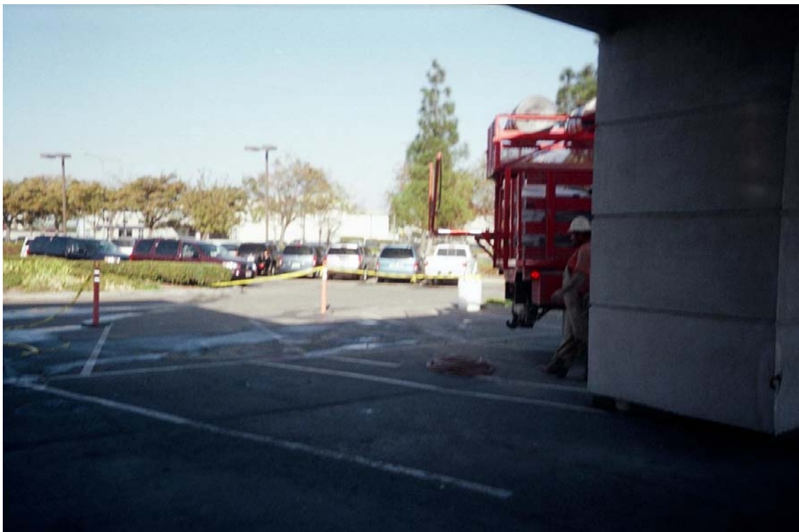
Photo 15: Work Area post drilling activities.
