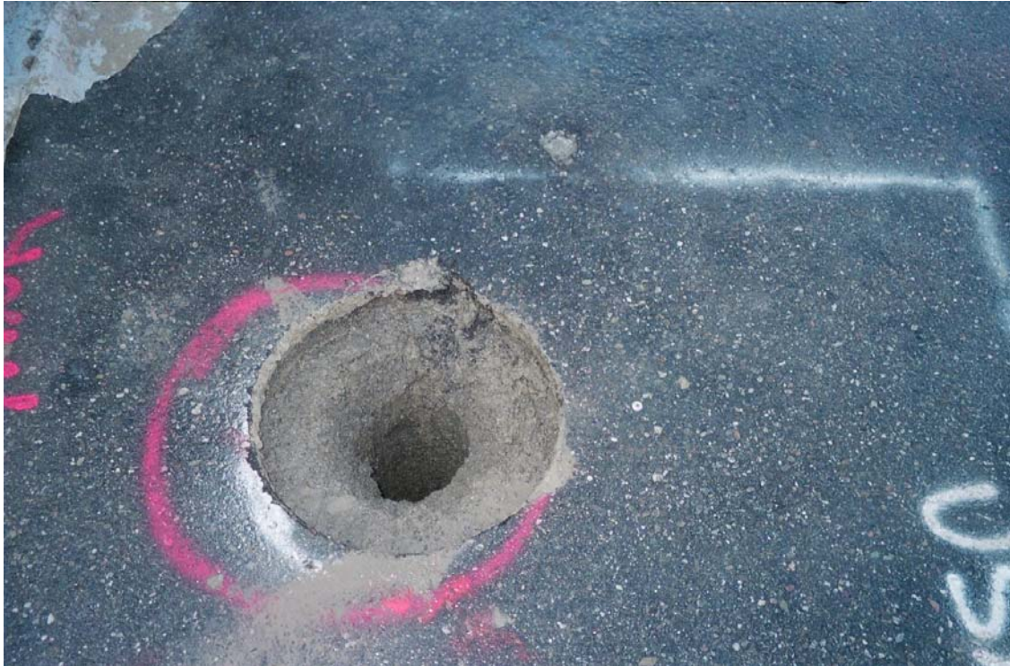
Photo 10: SB-VAS-a post drilling; pre concrete.
