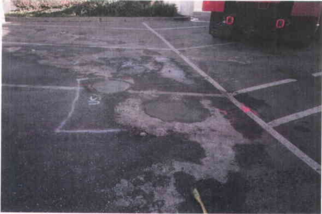
Photo 12: SB-9 and SB-VAS-1 Concrete Completion
