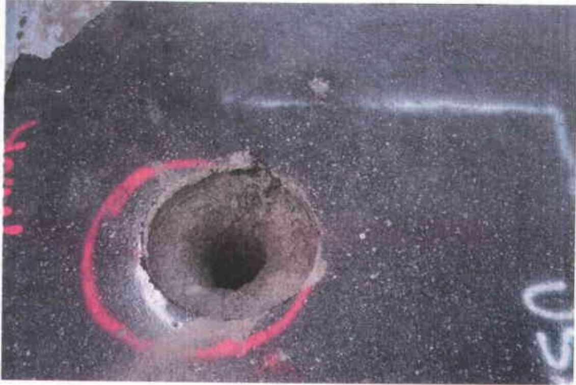
Photo 10: SB-VAS-a post drilling; pre concrete.
