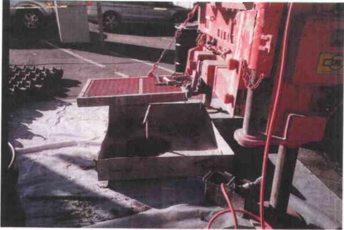
Photo 1: Hand auger to 5 ft bgs
