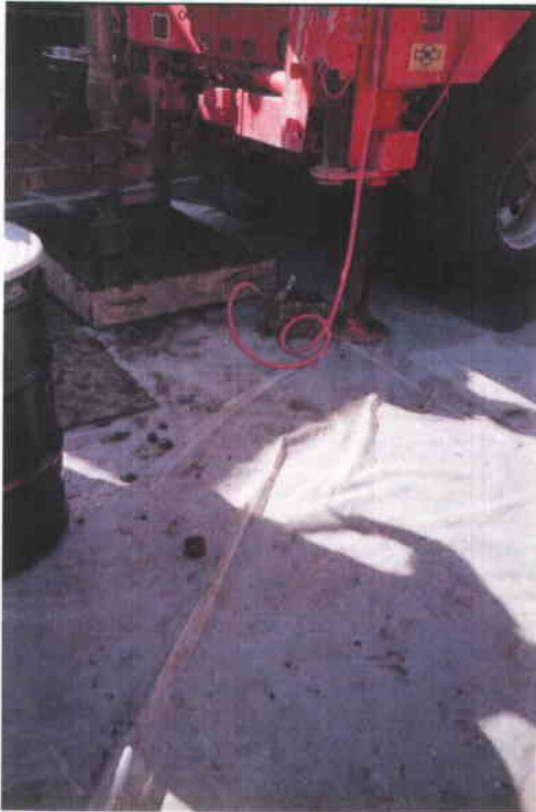
Photo 7: Drilling set up; with box to contain cuttings.
