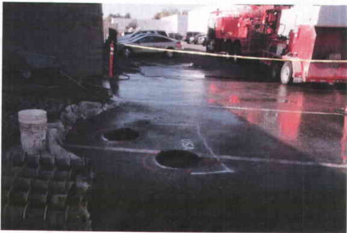
Photo 9: SB-VAS-1 and SB-9 post drilling, pre concrete.
