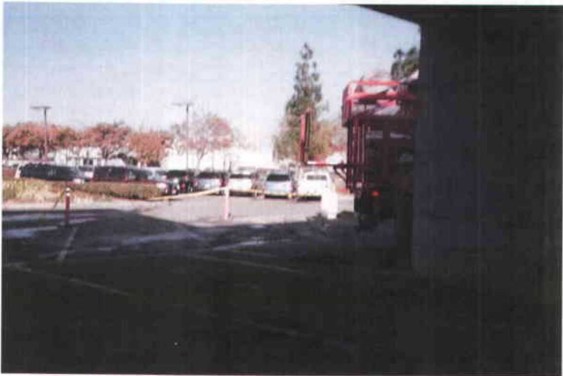
Photo 15: Work Area post drilling activities.
