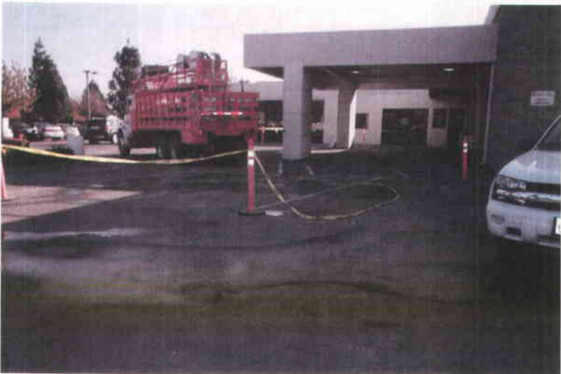
Photo 13: Work Area post drilling activities.
