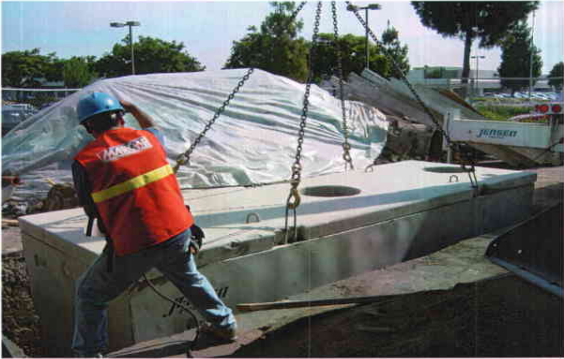
Photo #9: View of the Jensen 2,500-gallon OWS during installation.
