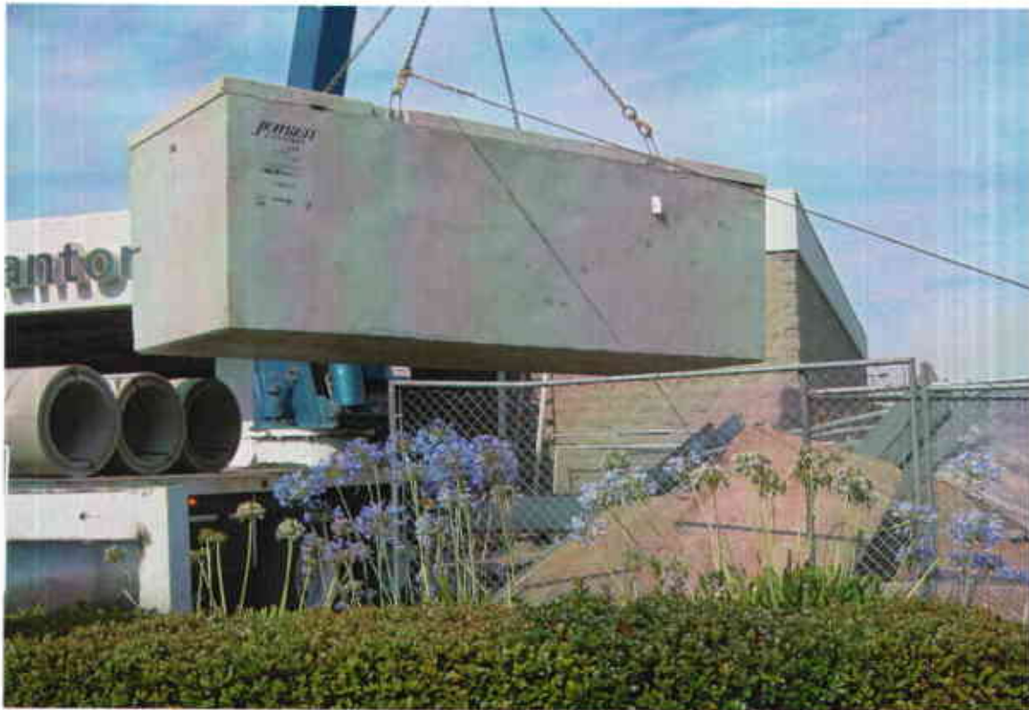
Photo #8: View of the new Jensen 2,500-gallon OWS during installation.
