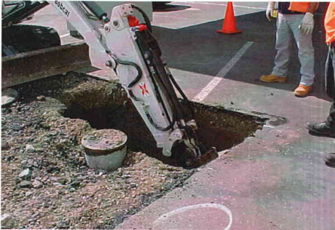
Photo #1: View of the initial excavation of the existing oil/water separator (OWS).
