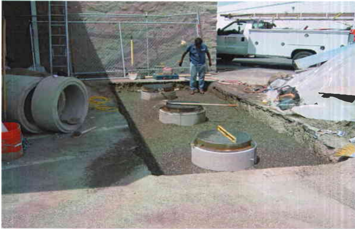
Photo #11: View of the entire OWS location following the OWS installation.
