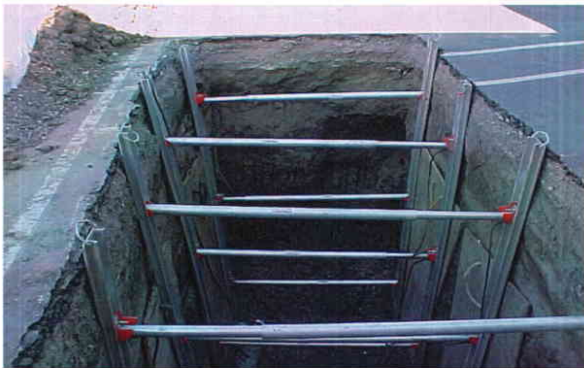
Photo #6: View of shoring placed in the OWS excavation.
