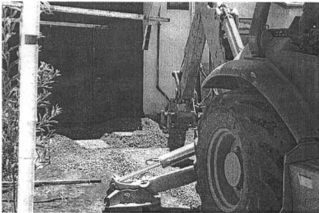
Final filling and compaction of outside excavation area.
