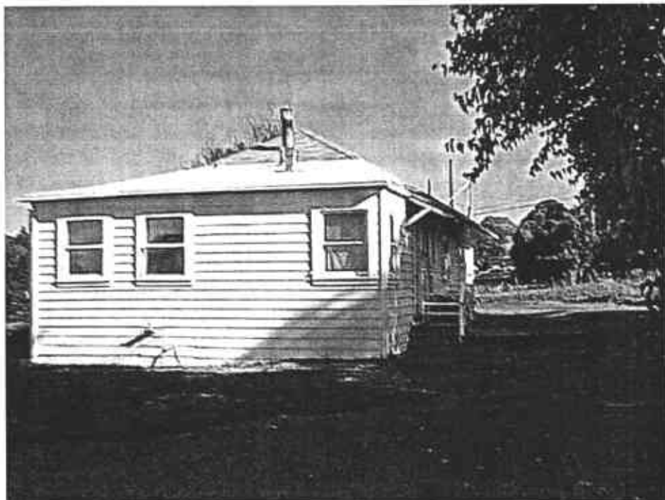
Figure 2B: Residence at 4611 Malabar Avenue, viewing north
