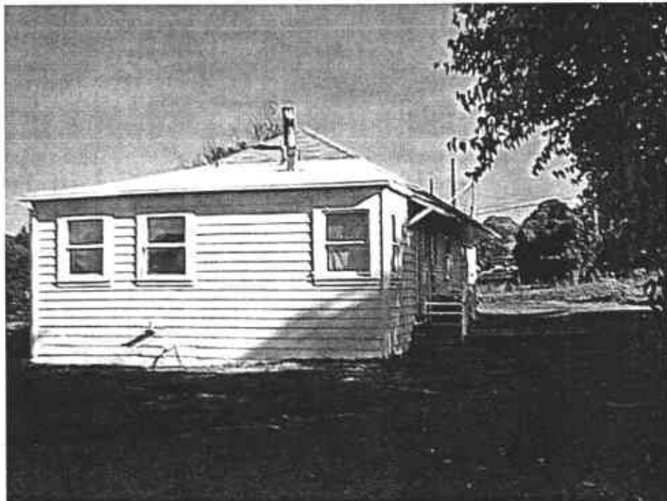
Figure 2B: Residence at 4611 Malabar Avenue, viewing north
