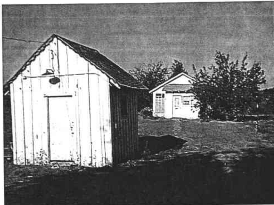
Figure 3B: 4605 and 4611 Malabar Avenue, viewing east
