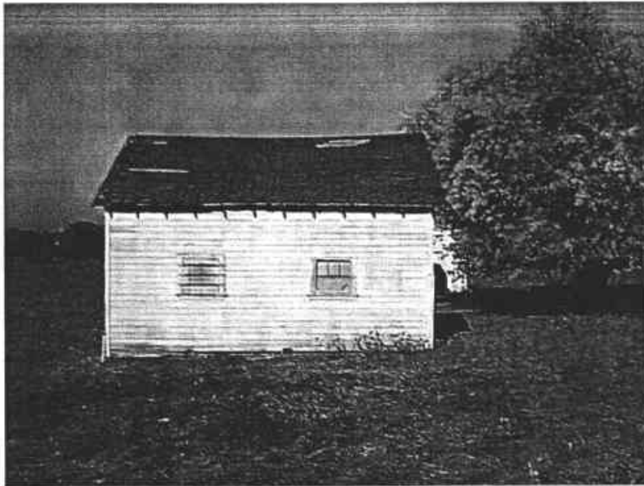
Figure 2A: Shed, viewing west
