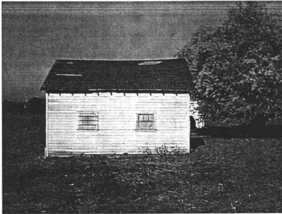
Figure 2A: Shed, viewing west
