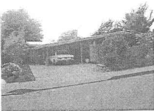
11-A: 18200 Block of Judy Street, West Side
