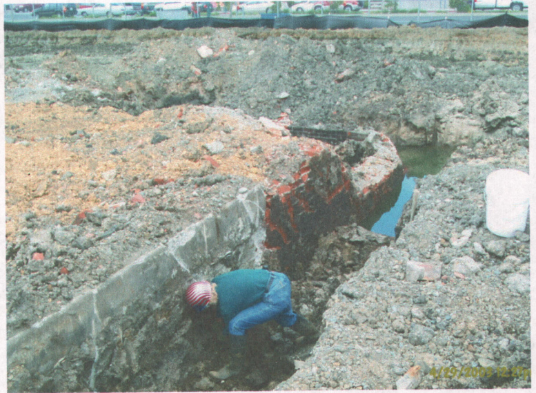
PIPING TRENCH SAMPLING
