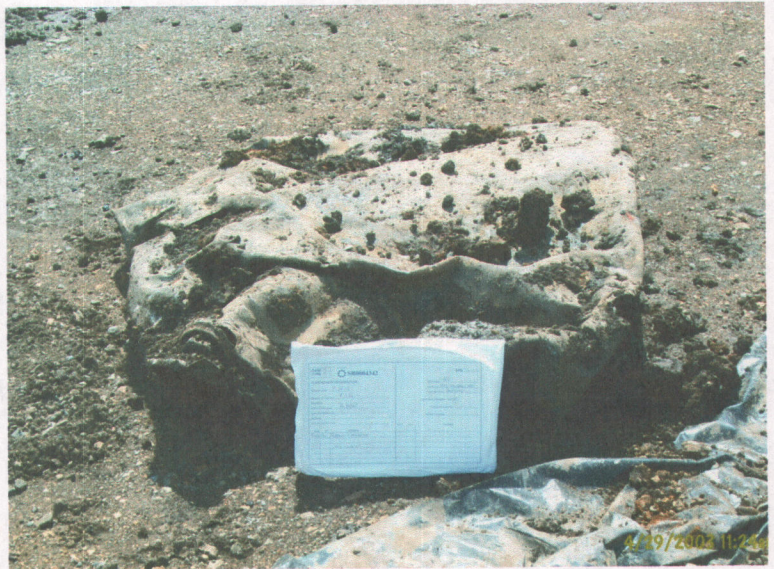
FORMER GASOLINE TANK FLATTENED W/ EXCAVATOR
