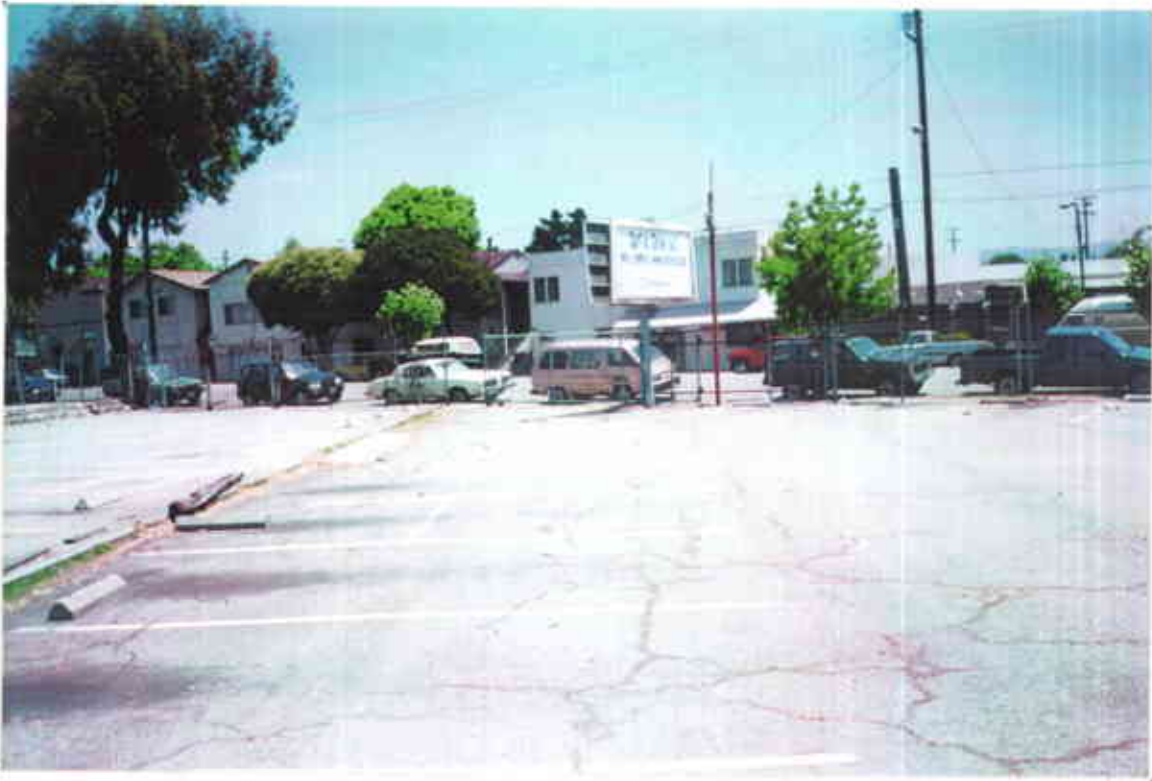
Plate 7: View east across Adeline Street.
