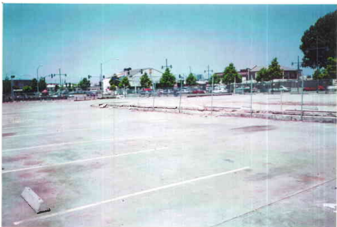
Plate 5: View across parking lot looking northwest
