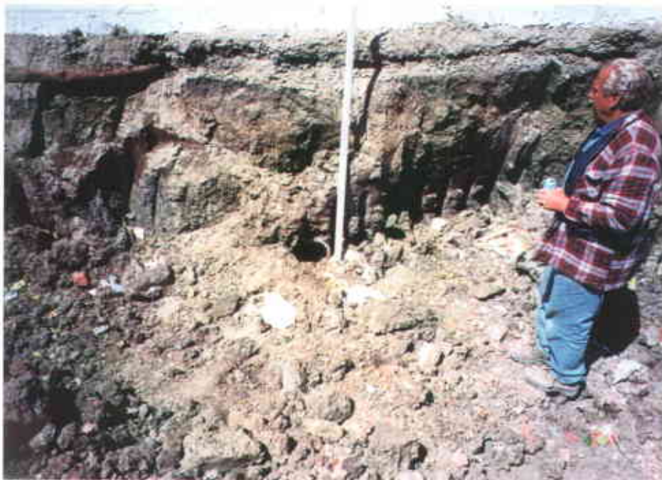
Plate 15: Sewer Pipe in West Wall of Remedial Excavation
