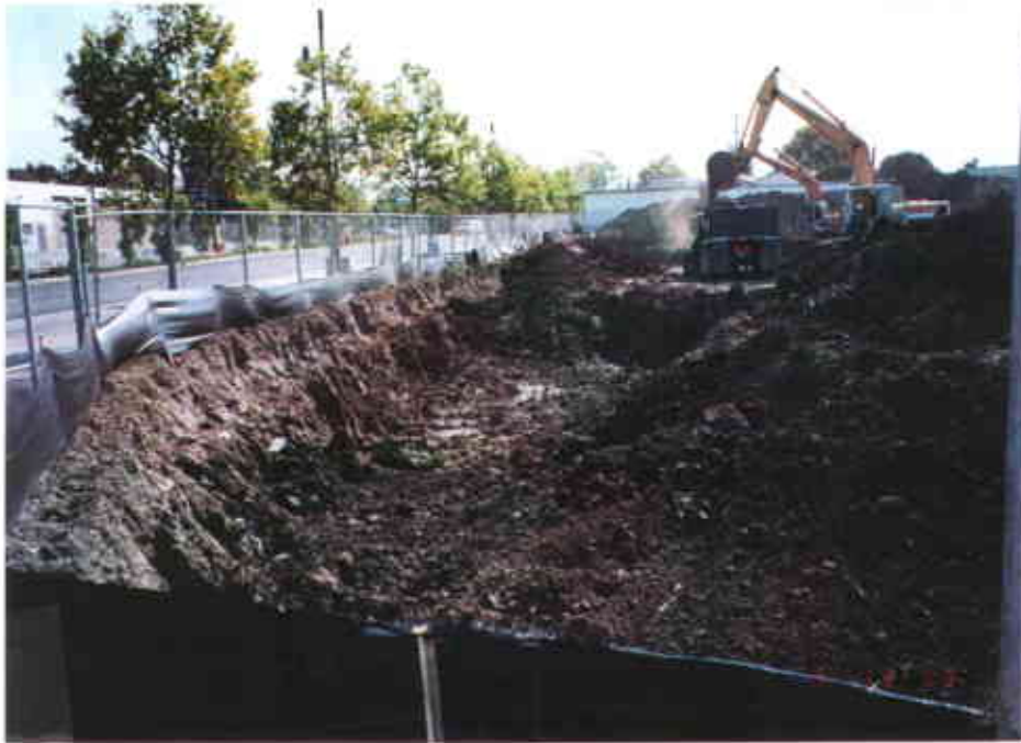
Plate 5: First Stages of Removal of Affected Soil Along 40th Street Frontage
