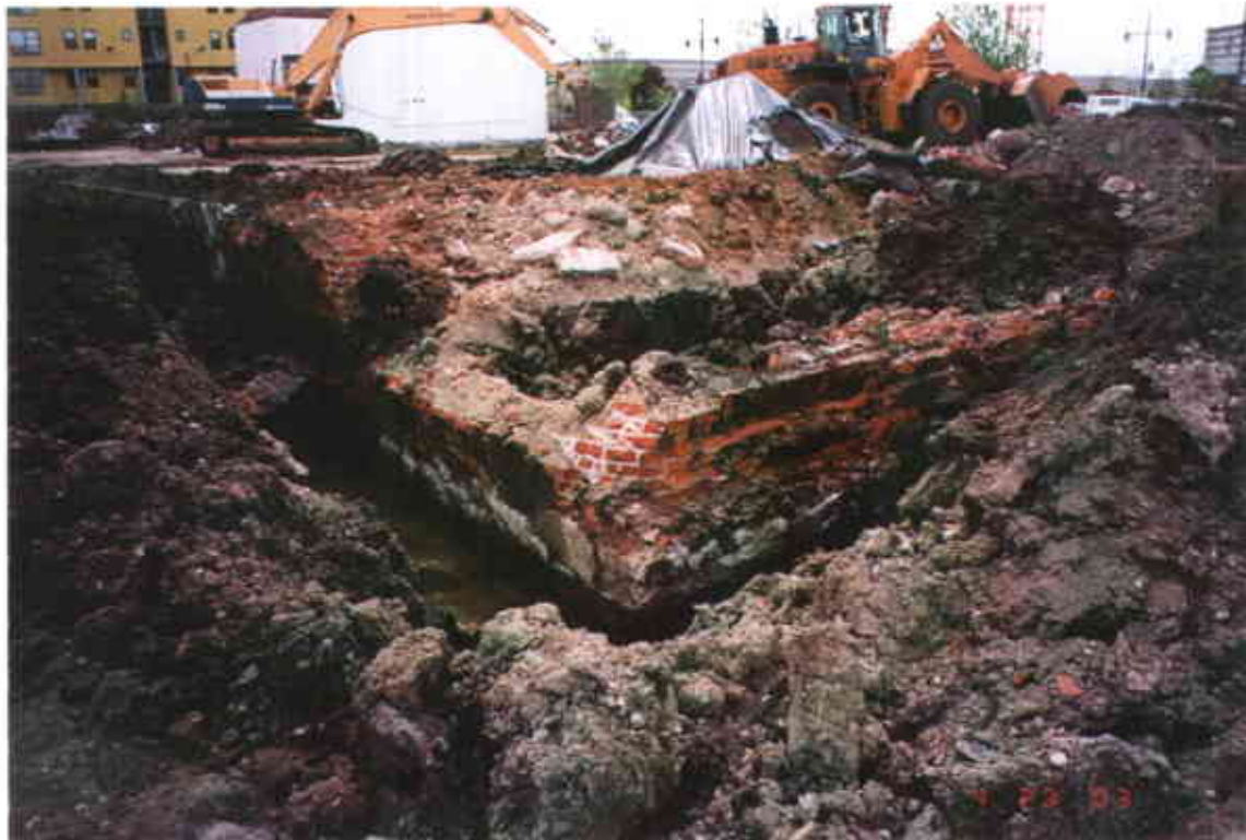
Plate 1: Example of Buried Mass Masonry Foundation Structures
