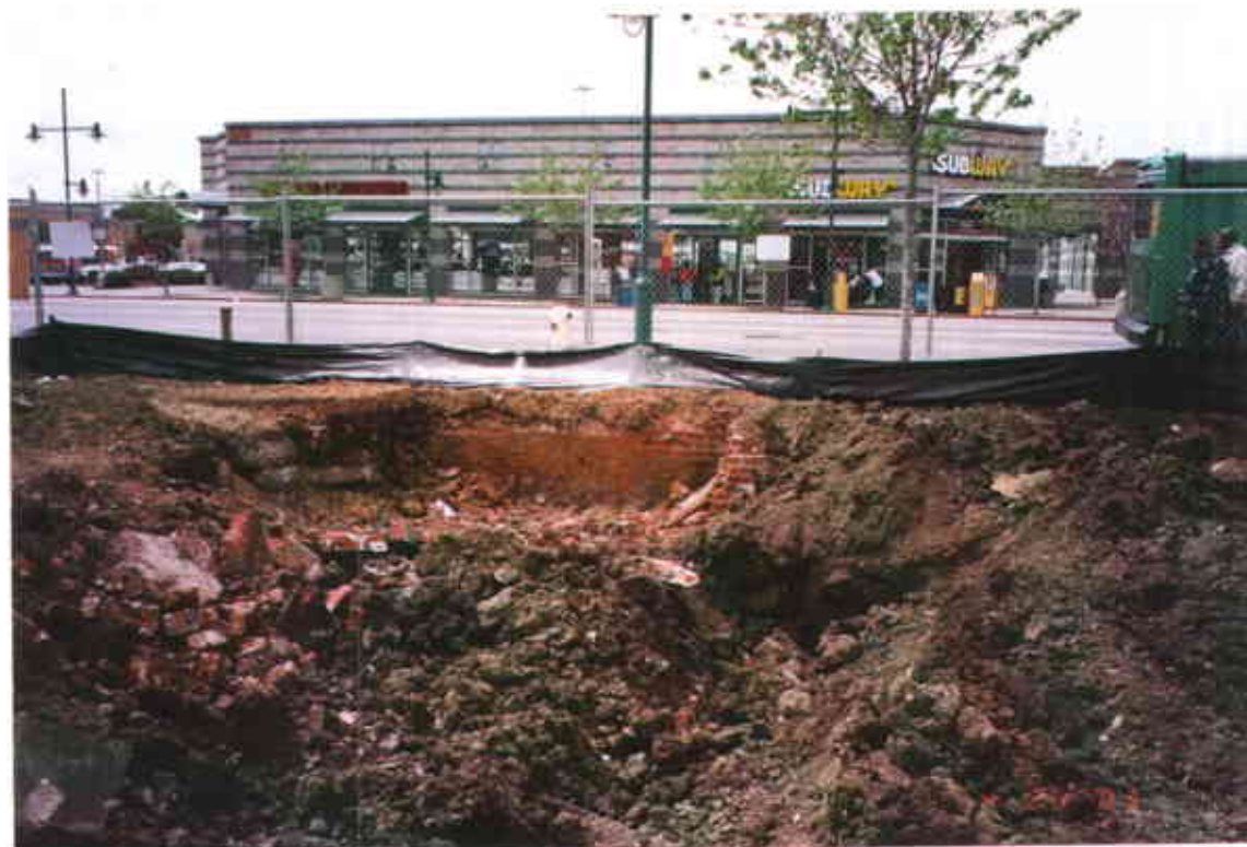
Plate 2: Exposed Basement Retaining Wall Along San Pablo Avenue Frontage
