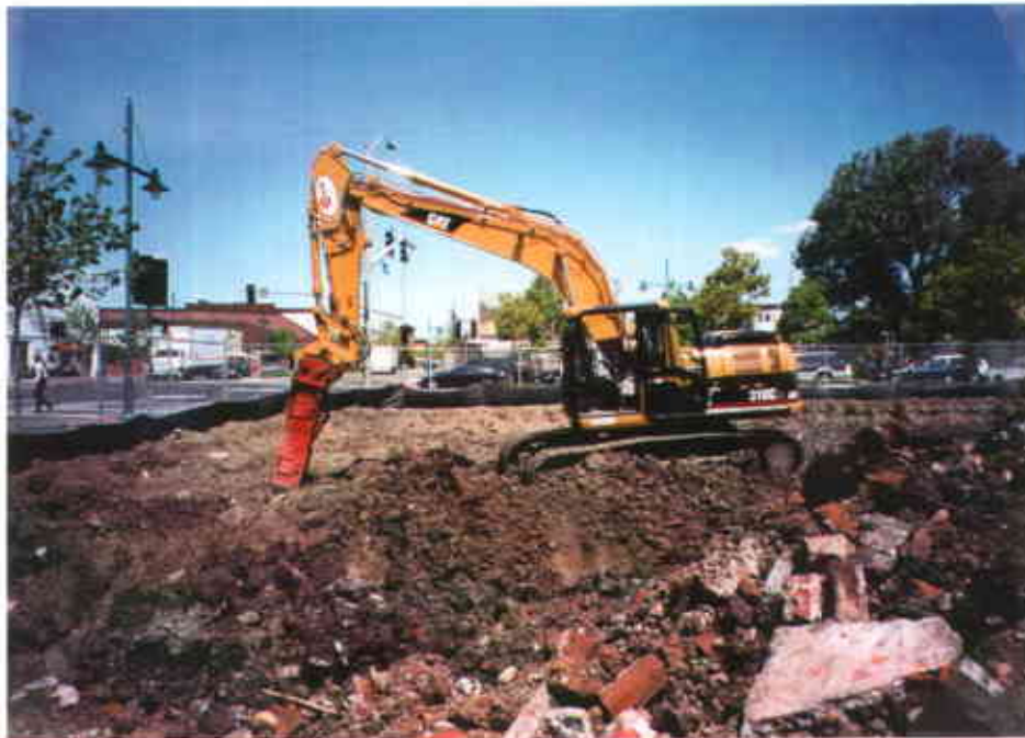
Plate 4: Hydraulic Breaker Demolishing Buried Masonry and Concrete
