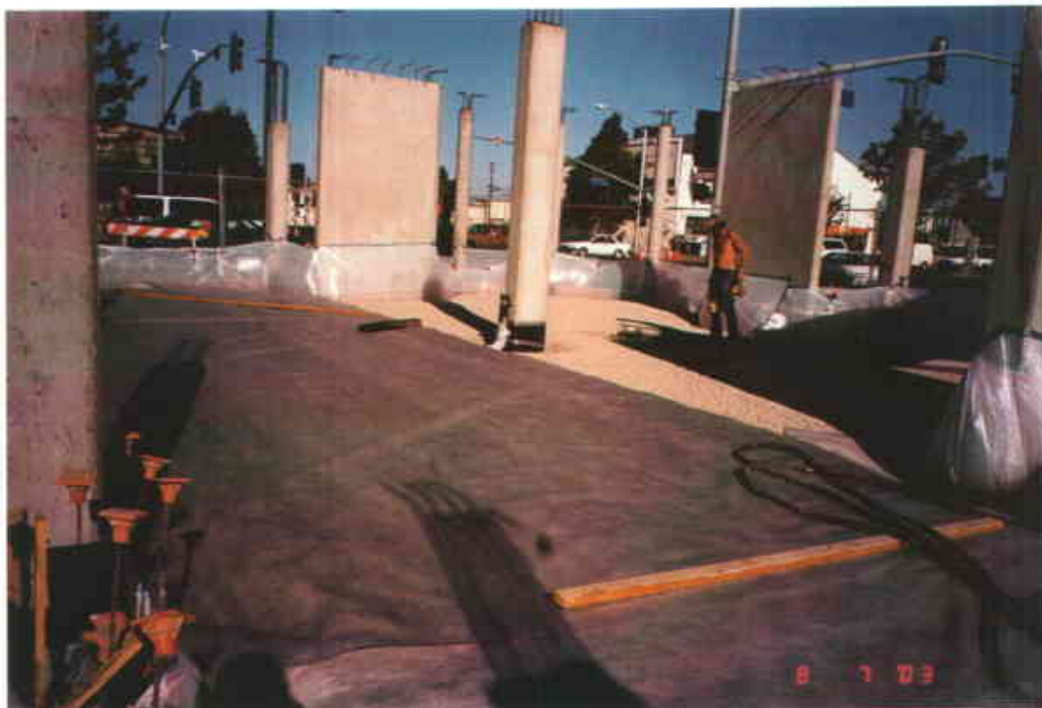
Plate 18: Geotextile Fabric Laid Down to Receive Liquid Boot ® Membrane
