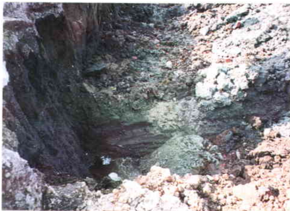
Plate 8: Streambed Deposits Exposed in Western Wall of Remedial Excavation
