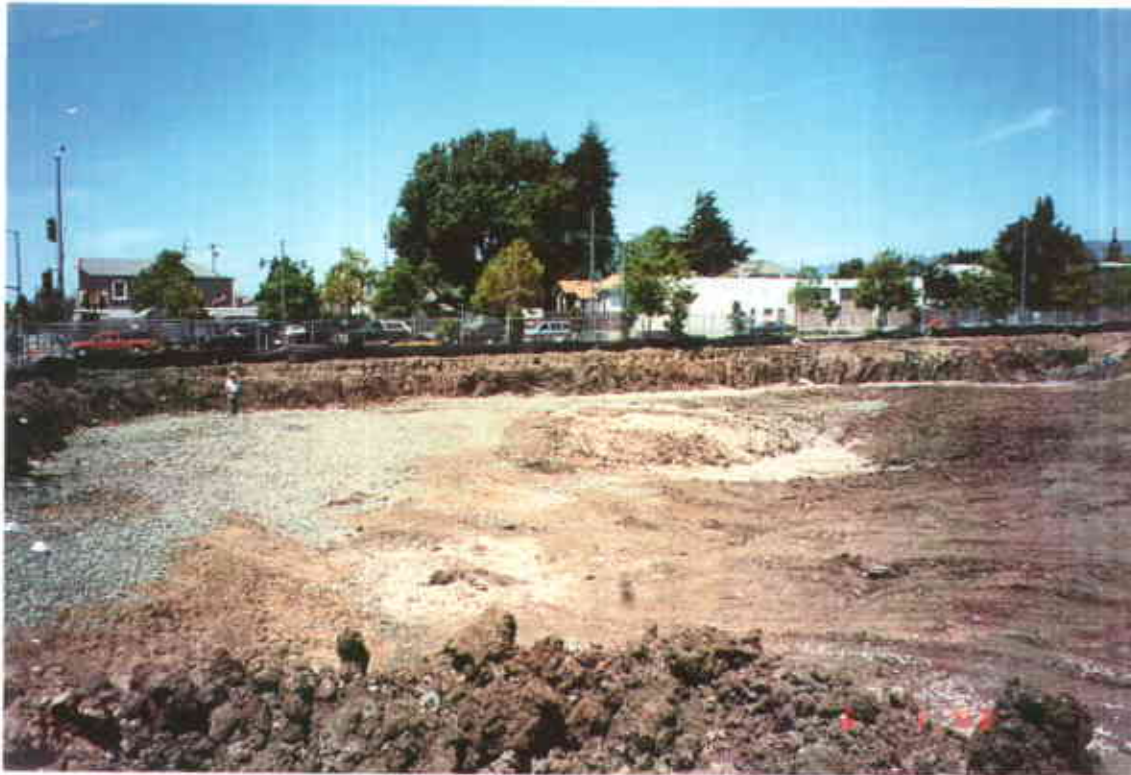
Plate 14: The Remedial Excavation Viewed from the South
