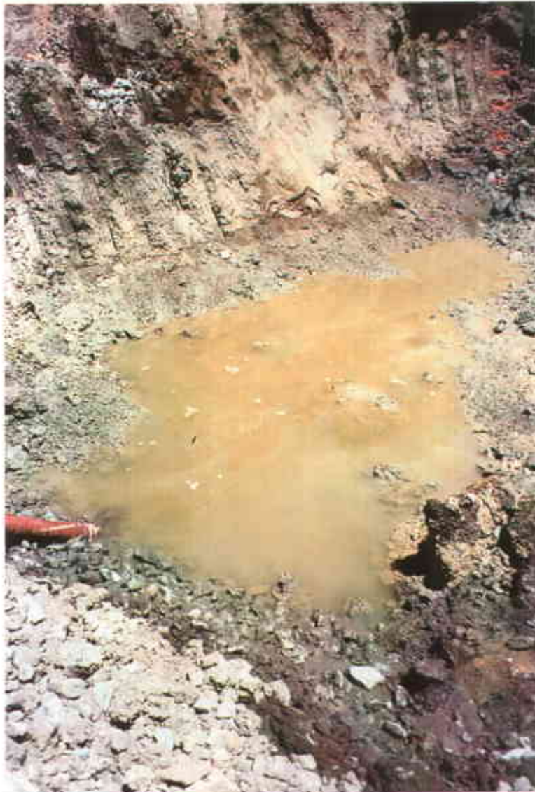
Plate 11: De-watering Paleo Streambed Excavation to Permit Placement of Clay Cap
