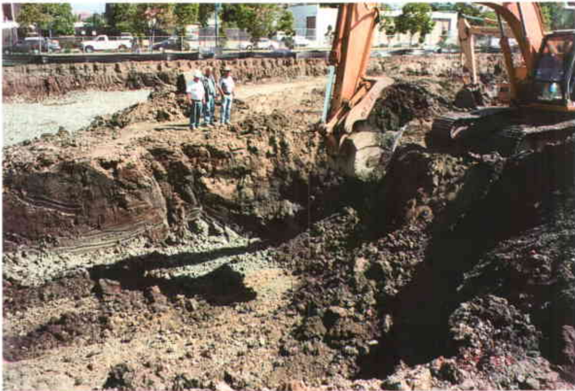
Plate 9: Excavation to Remove Paleo Streambed Deposits
