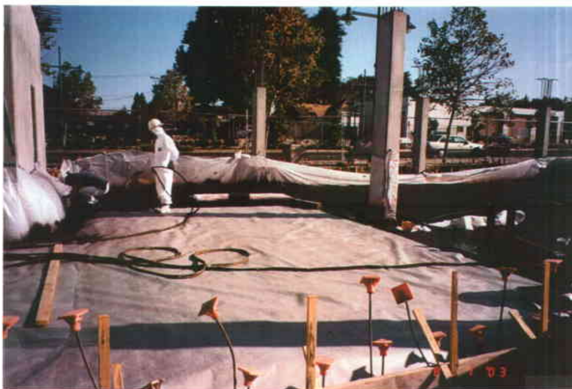
Plate 19: Application of Liquid Boot ® Membrane
