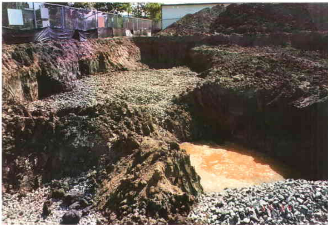
Plate 7: Typical Excavation Cell
