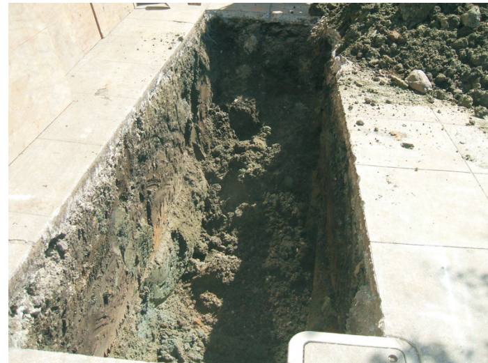
PHOTO 4: UST EXCAVATION CAVITY LOOKING EAST FROM WEST END OF EXCAVATION.
