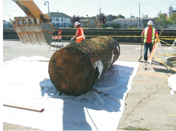
PHOTO 2: PREPARING TO CLEAN UST PRIOR TO LOADING ONTO TRUCK.
