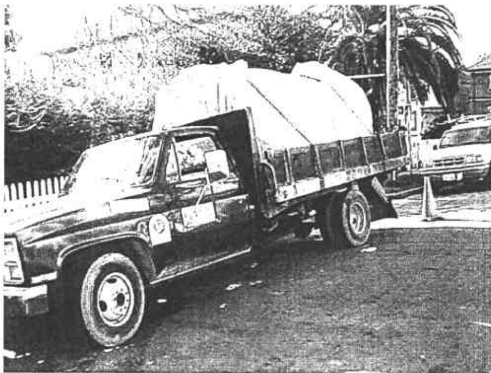
Tank loaded on truck and ready for transport and disposal
