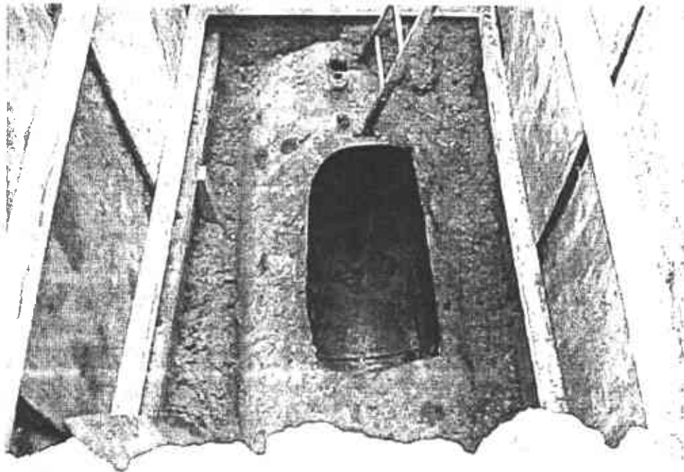
Tank in excavation ready for removal
