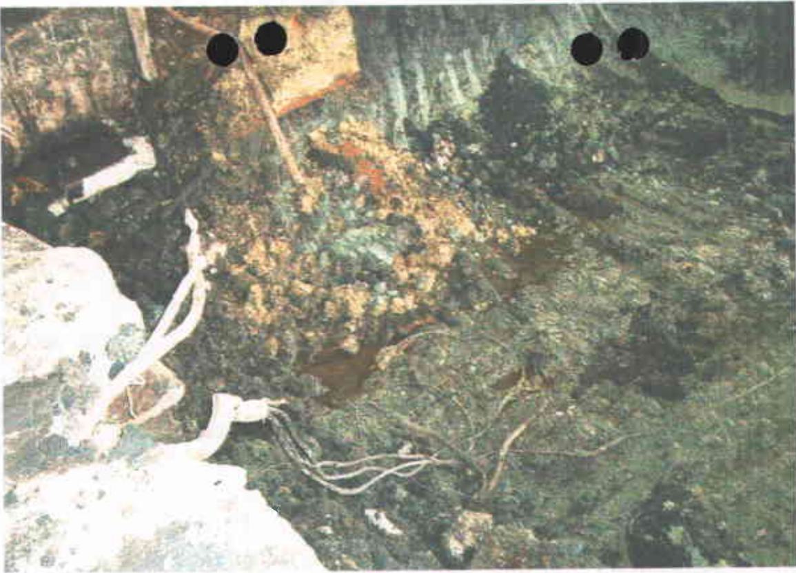
Photograph 5 – Bottom & sidewall near northwest corner of excavation.
