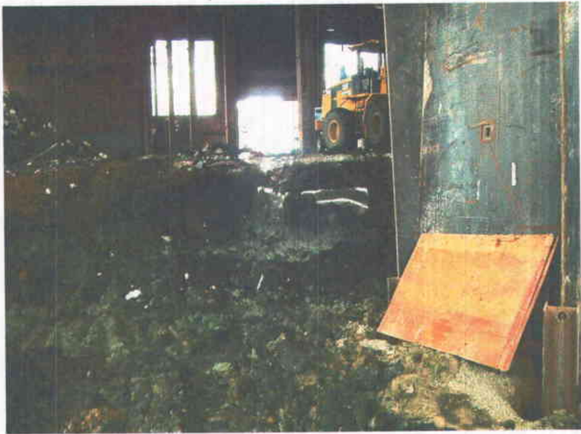
Photograph 2 –View of west side of excavation sidewall.
