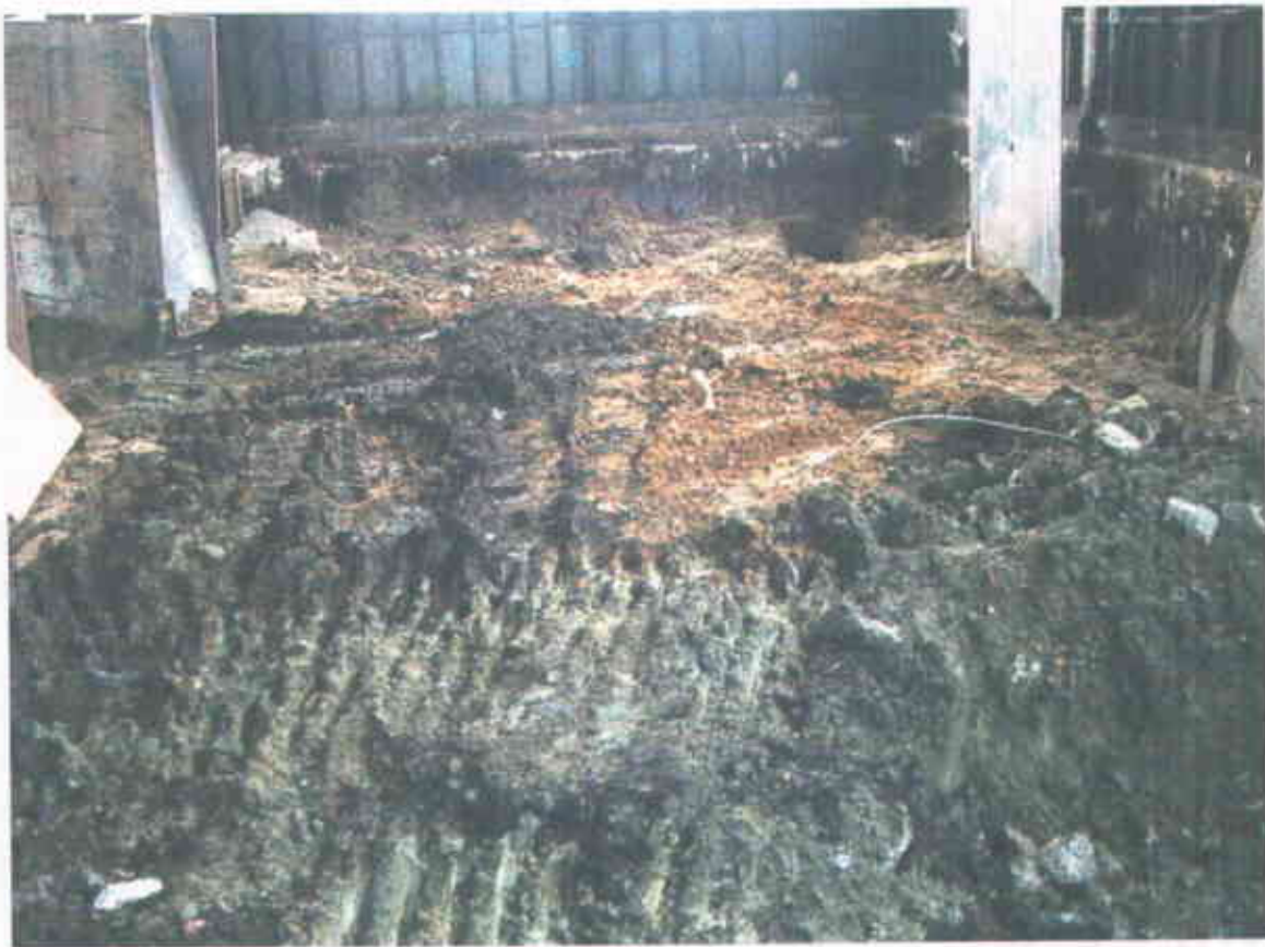
Photograph 6 – Overall view of excavation.
