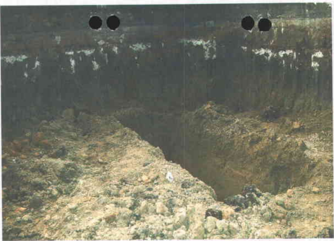
Photograph 1 – Southeast corner of building
