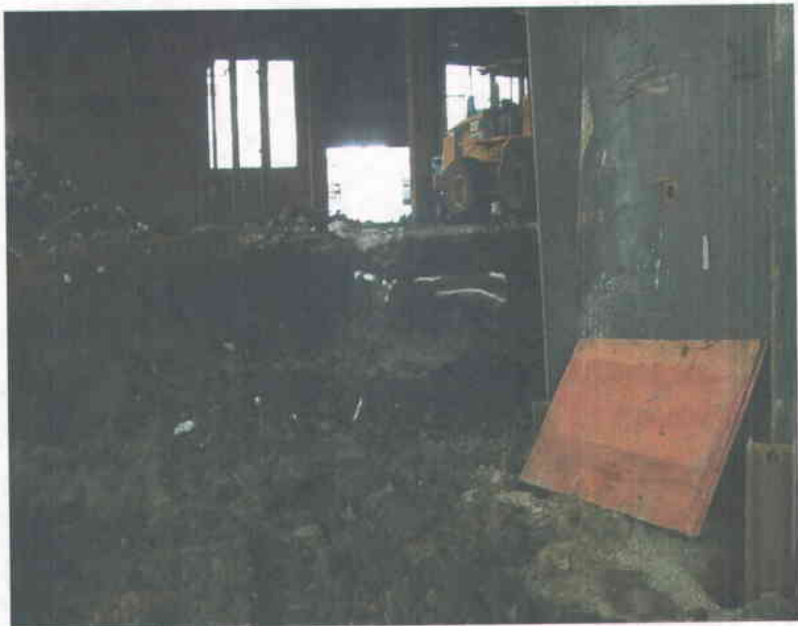
Photograph 4 – View inside excavation green contaminated soil, black & tan native.
