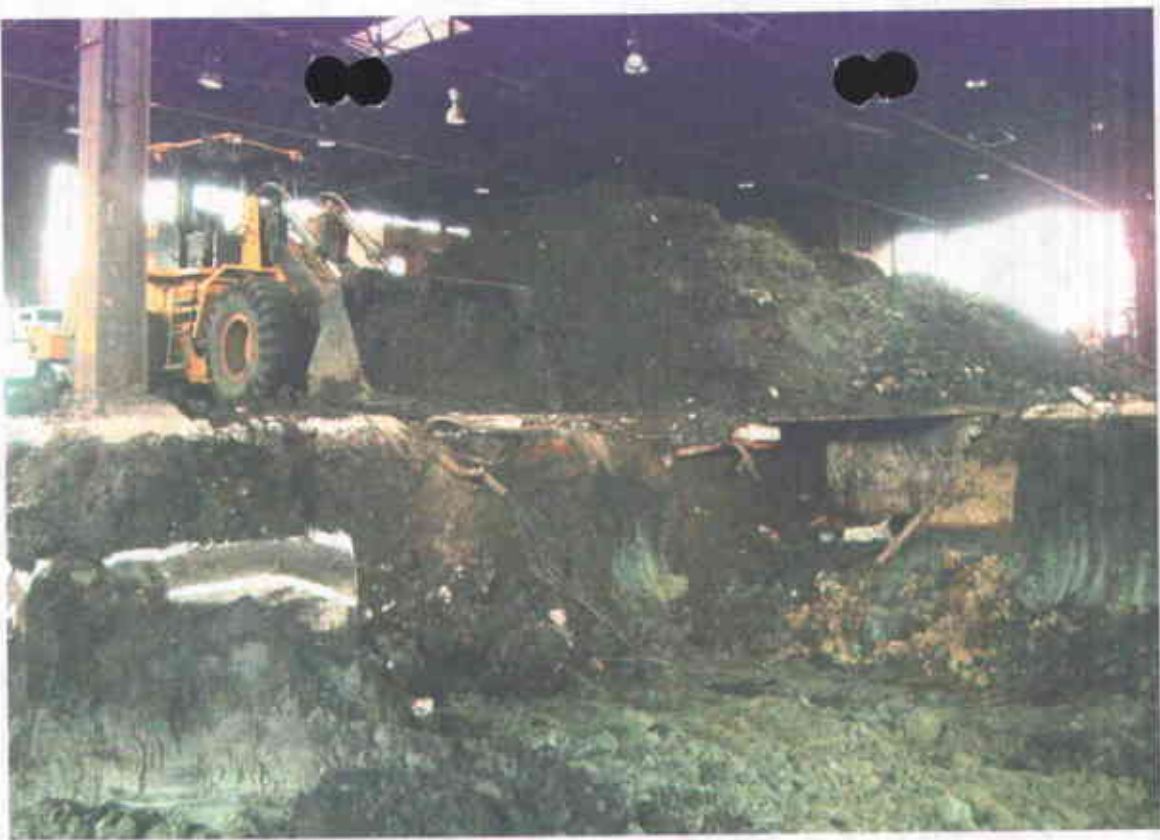
Photograph 3 – Northwest corner of excavation.
