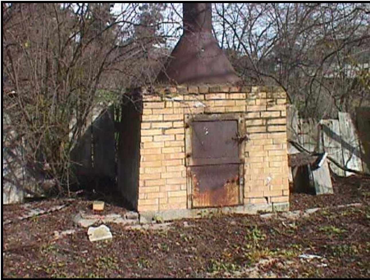
Former Incinerator – Friesman Ranch Property, Livermore, CA
