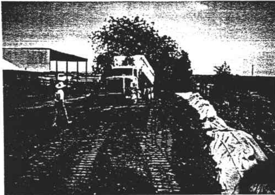
SOIL STOCKPILE LOOKING EAST.
