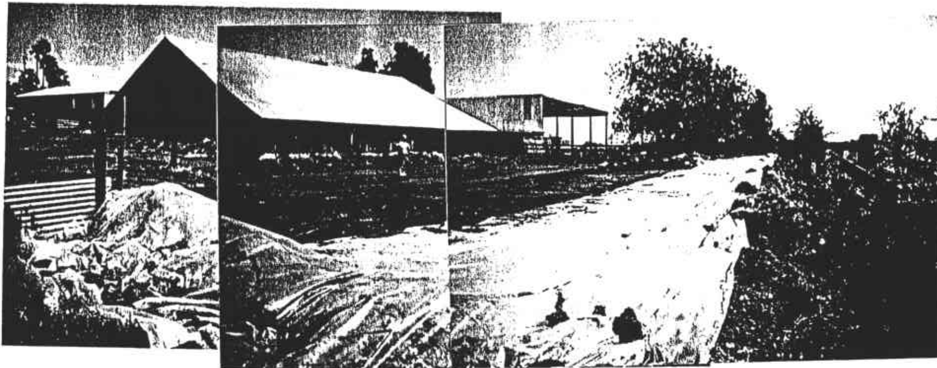
SOIL STOCKPILE LOOKING EAST. NOTE: VISQUEEN SHEETING ON SURFACE.
