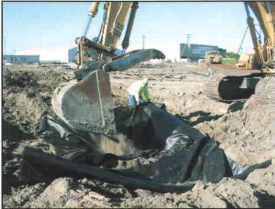
Photo #17: Backfilling foundation pile excavations.
