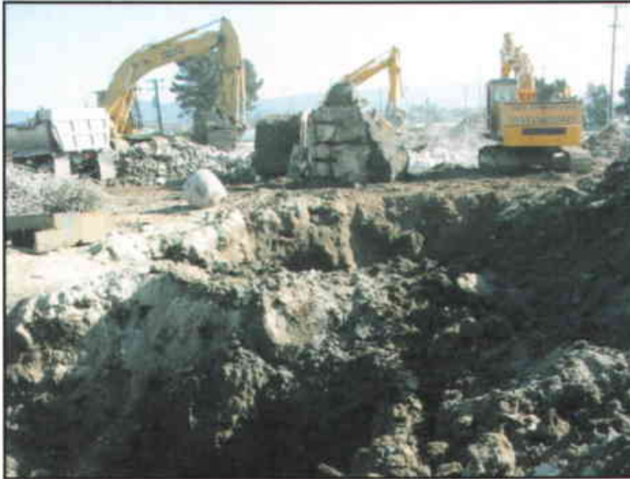
Photo #13: Belowground structures, including sumps and pits, were removed and demolished.
