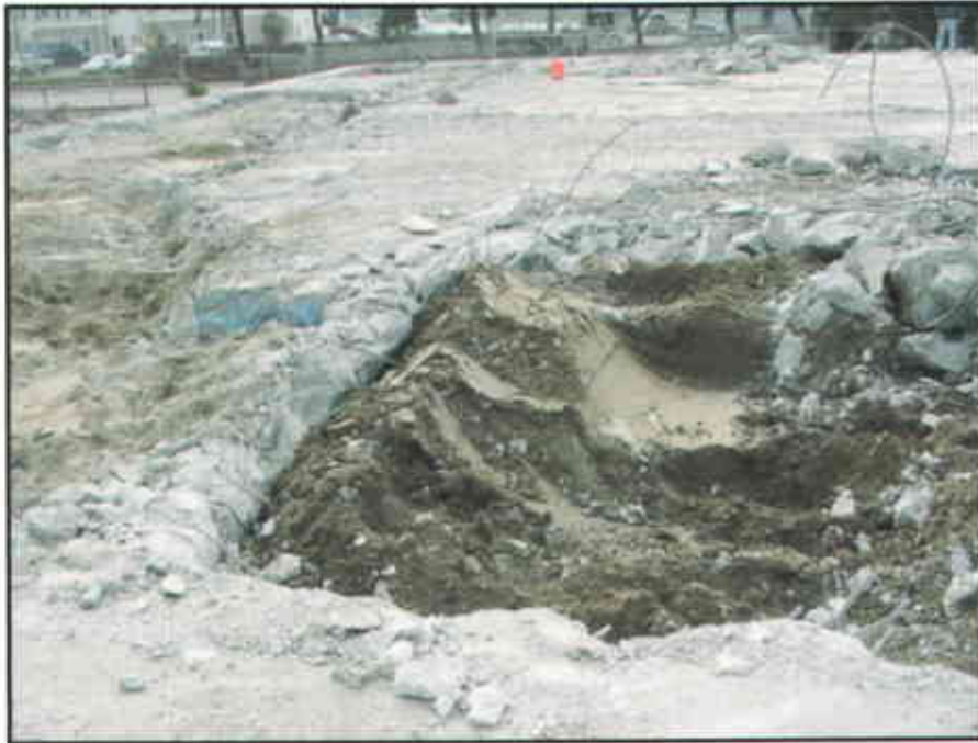
Photo #7: Sand fill was located along the eastern edge of the Building 1 foundation. Soil fill was located throughout the remainder of the Building 1 foundation.
