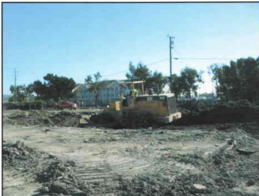
Photo #18: Compaction using a bulldozer equipped with sheepfoot wheels.
