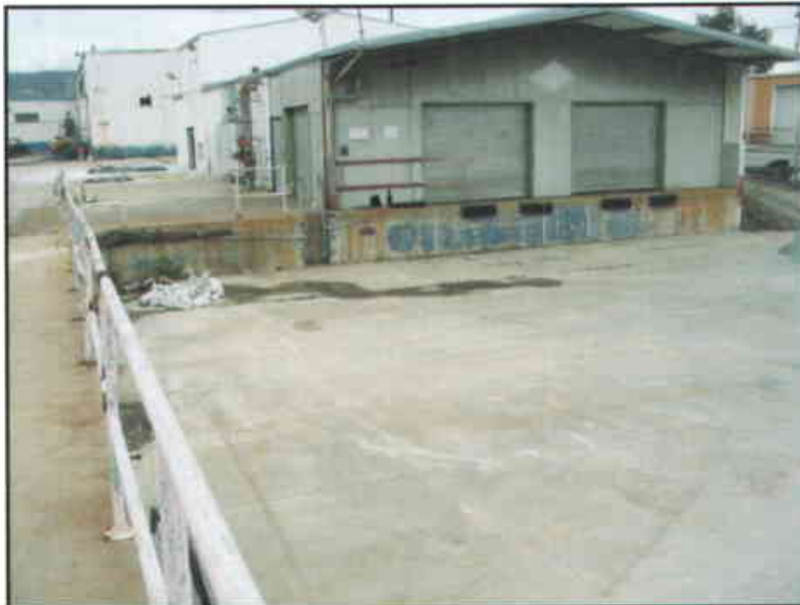
Photo #2: Building 2 and loading area prior to demolition activities.
