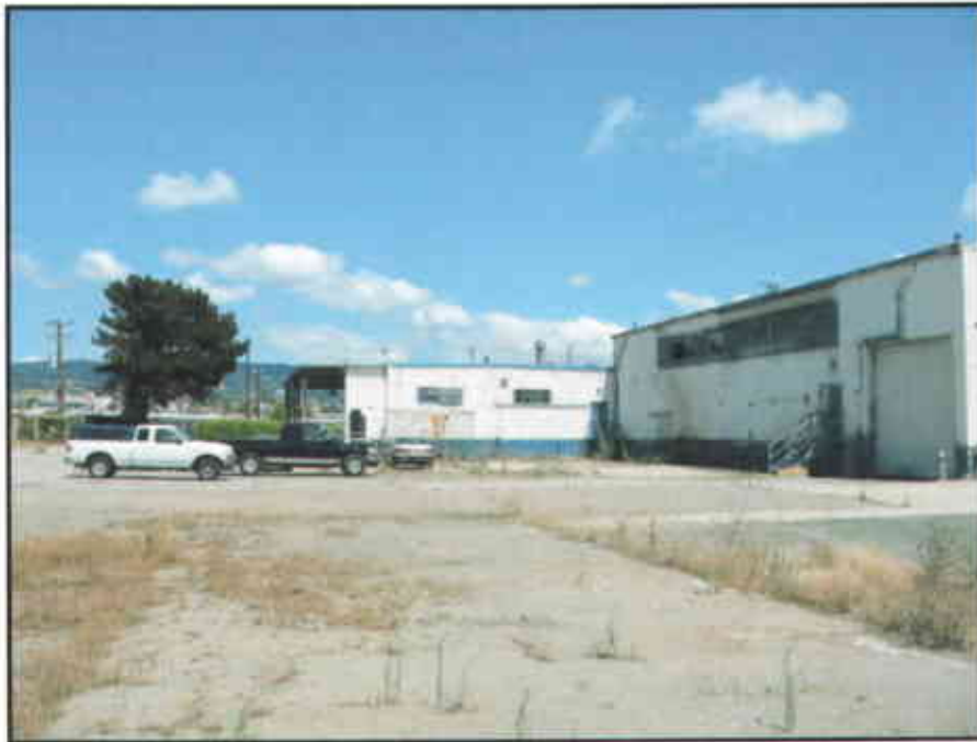
Photo #1: Building 1 and loading area prior to demolition activities.
