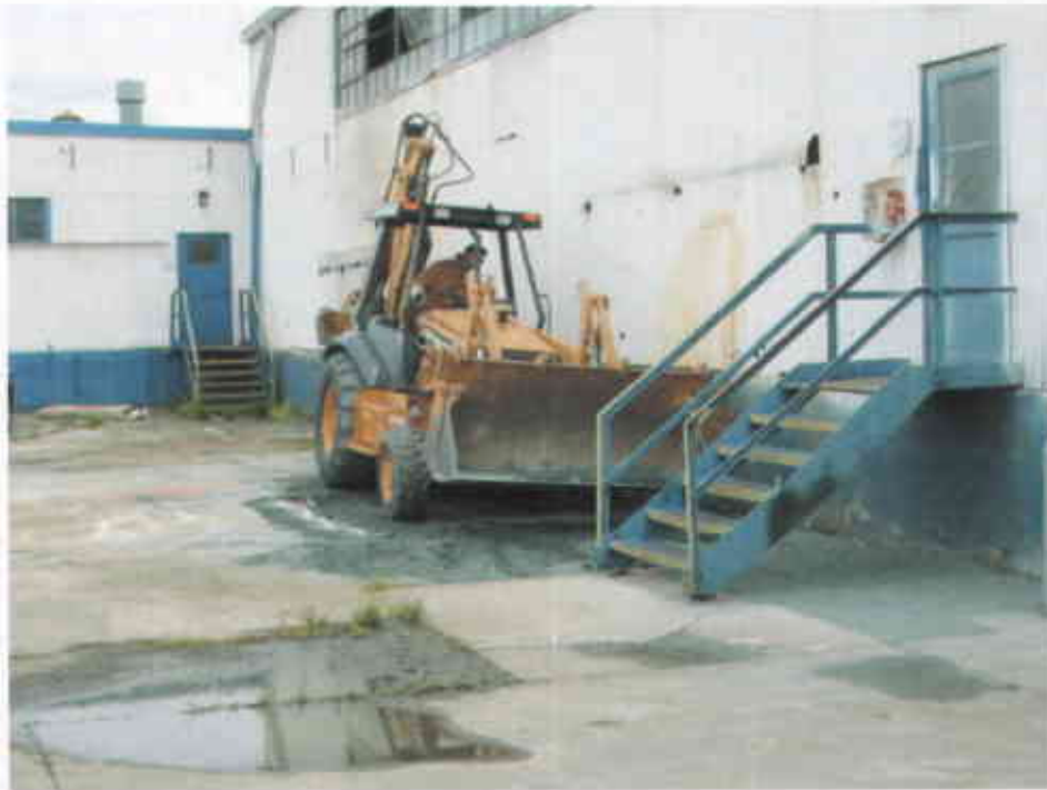
Photo #12: Compaction of backfill near Boring KB-13.
