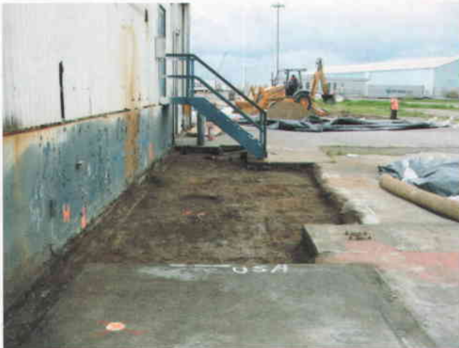
Photo #6: Excavation of soil near Boring KB-13 complete.
