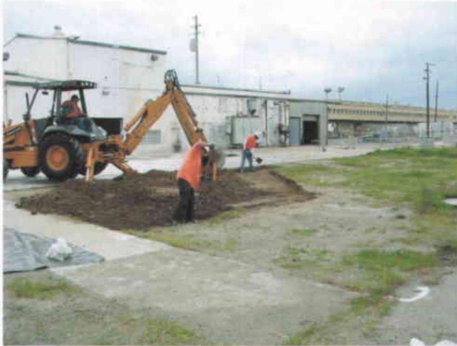
Photo #3: Excavation in progress at Boring KB-11.
