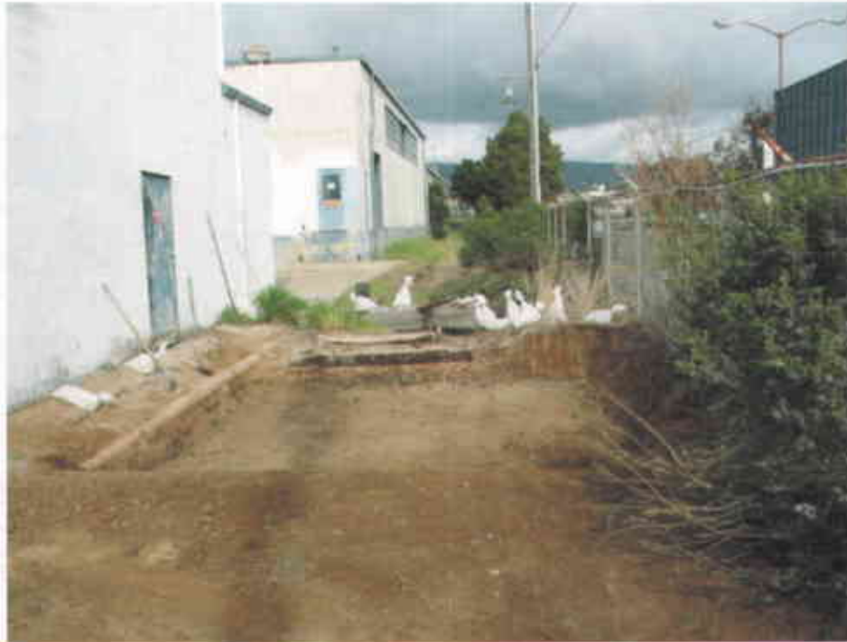
Photo #1: Excavation of soil at Boring KB-7 complete.
