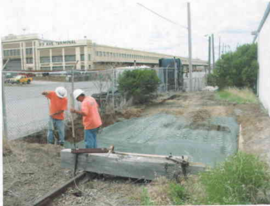
Photo #8: Placing backfill at excavation for Boring KB-7.
