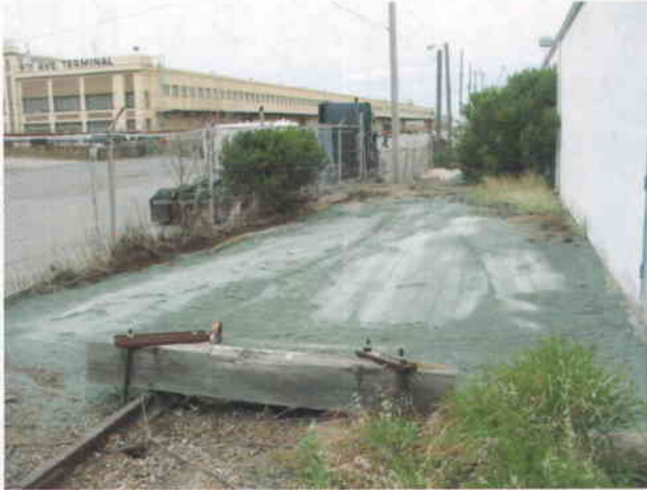
Photo #9: Backfill complete at excavation for Boring KB-7.
