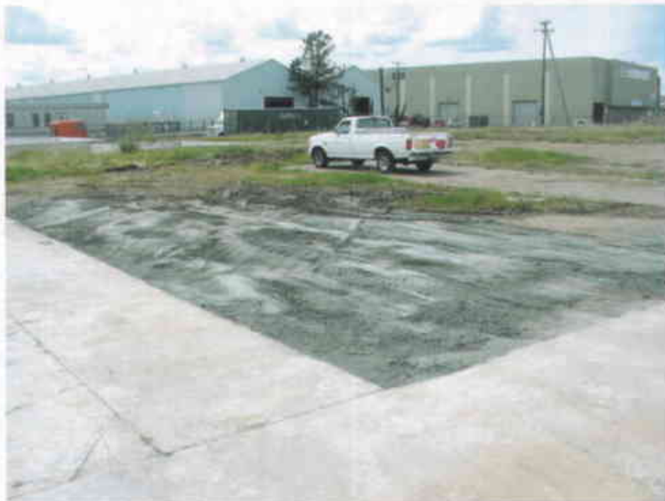
Photo #10: Backfill complete at excavation for Boring KB-11.
