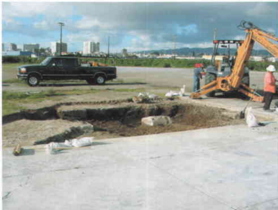
Photo #4: Excavation of soil at Boring KB-11 complete.
