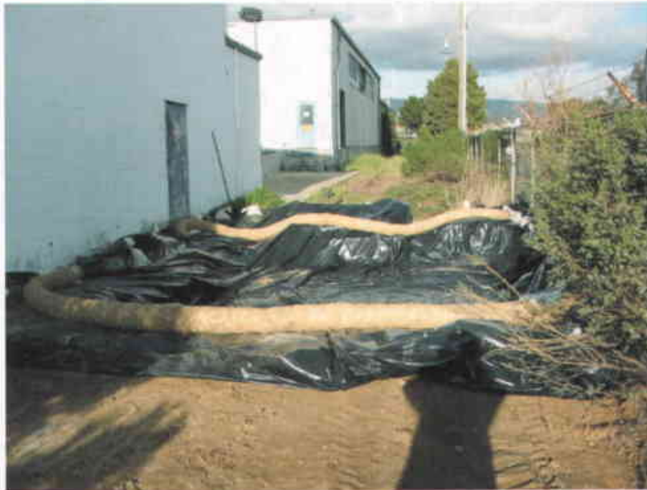
Photo #2: Excavation at Boring KB-7 lined with plastic.
