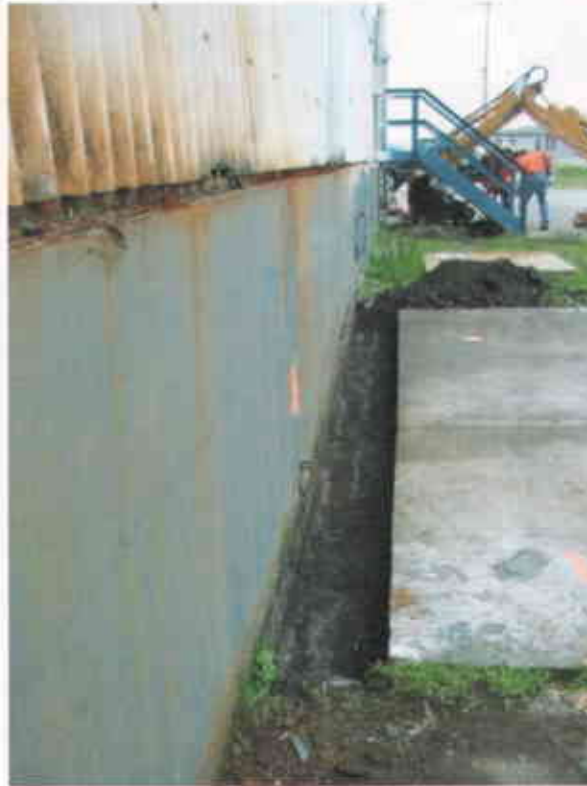
Photo #5: Start of excavation, including hand shoveling, near Boring KB-13.
