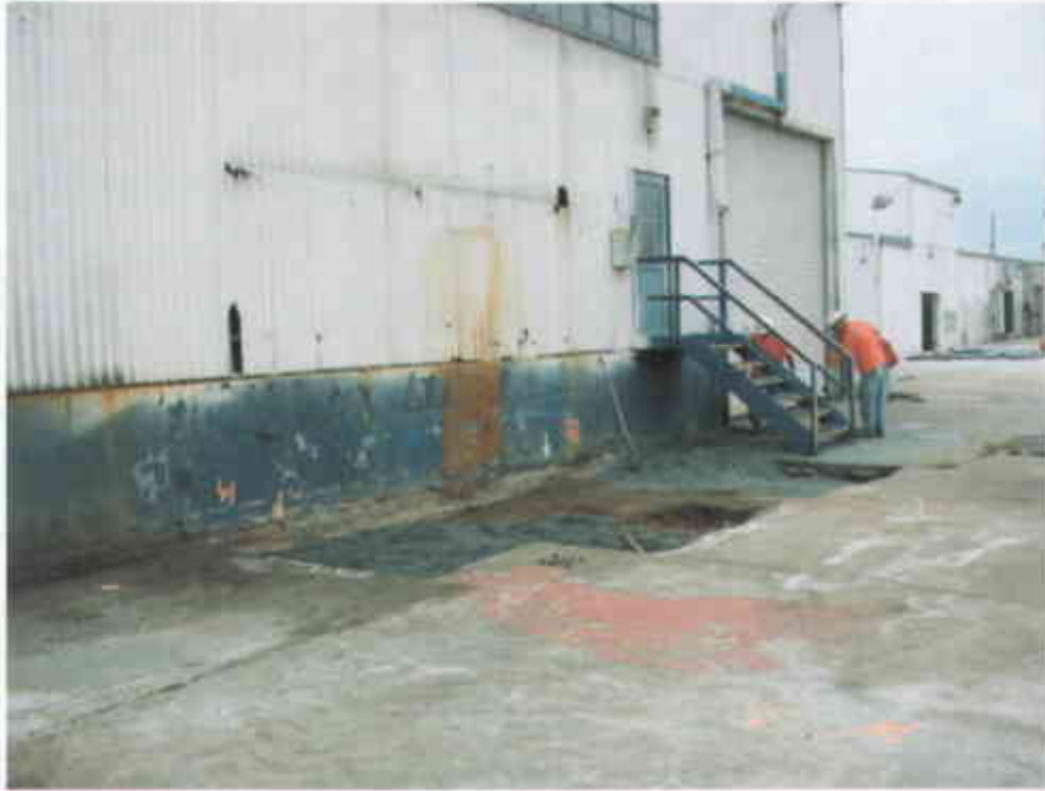
Photo 11: Placing backfill at excavation near Boring KB-13.
