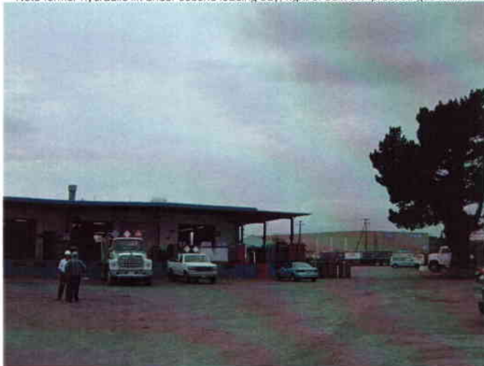
Photo #2: View looking west at front right loading docks of Building One. Beige building in right background is furniture warehouse beyond property boundary along 9 th Avenue at Defremery Avenue..
