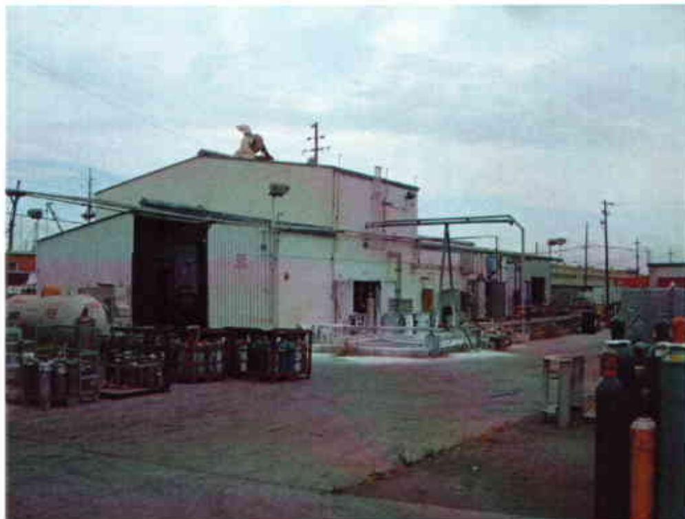
Photo #12: View looking south at acetylene generation and bottling works at Building Two. Underground concrete sludge pit showing signs of spillage in center, right side of building.
