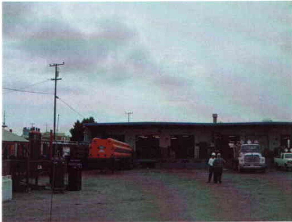
Photo #1: View looking southwest at front left loading docks of Building One at 901 Embarcadero. Utility pole and transformer at approximate southeastern property boundary along 10 th Ave. Note former hydraulic lift under second loading bay, right of bulk compressed gas trailer.
