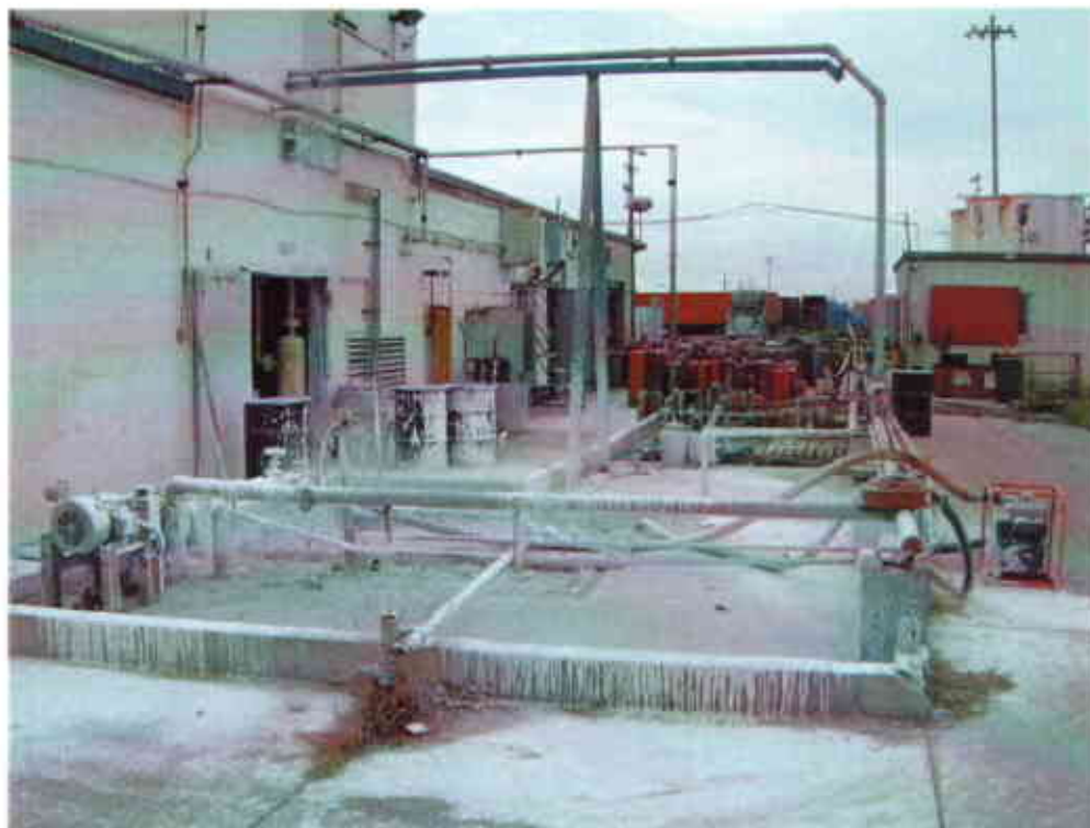
Photo #15: View looking southwest at underground concrete sludge pit on north side of Building Two, outside of acetylene reactor room with open doors. Note spillage and use of trash pump at far right.
