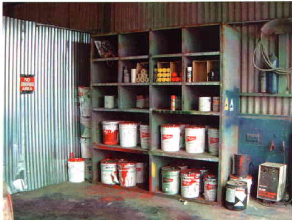
Photo #10: View of cylinder paints located adjacent to paint spray booth on southwest end of Building One. Black five-gallon can of paint in lower right labeled as "marine pollutant."
