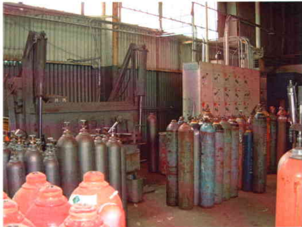
Photo #8: Bead blast cylinder paint remover on left, aged electrical circuit breakers to right along northern wall of southwestern end of Building One.
