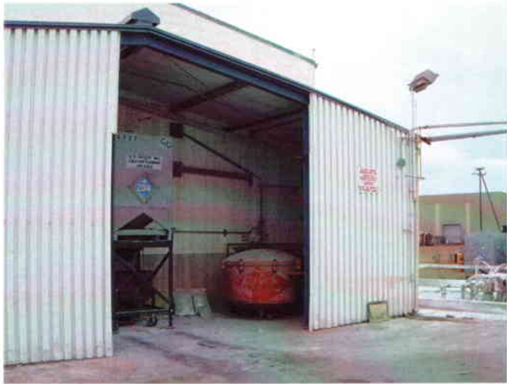
Photo #13: View looking west at east end of Building Two with bottom-emptying calcium carbide bin on stand in center. Squat red vessel on right is "monkey dust"-containing acetylene purifier.
