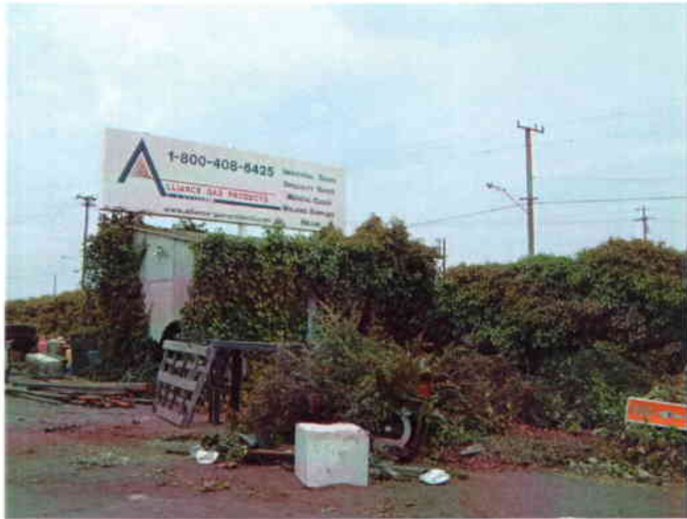
Photo #3: View looking northwest at frontage billboard for Praxair sub-tenant, Alliance Gas Products, along Embarcadero (Behind ivy covered fence). Small amount of miscellaneous solid waste in front of former vehicle maintenance shed with transite-asbestos sheet covering
