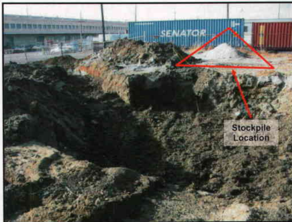
Photo #3: Lime-Impacted Soil at Ground Surface within the Footprint of the Former Containment Berms of the Lime/Water Decant Tanks
