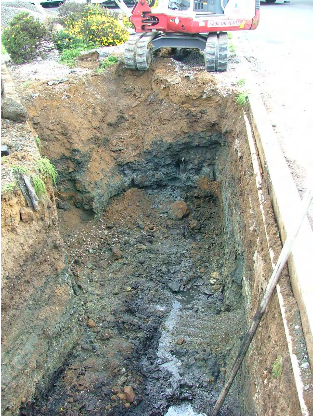
Picture 4: Initial excavation 2/12/2009
