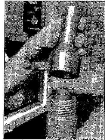
Figure 4.26. Place a drive bumper on top of the inner rods and thread a drive cap onto the outer casing.
