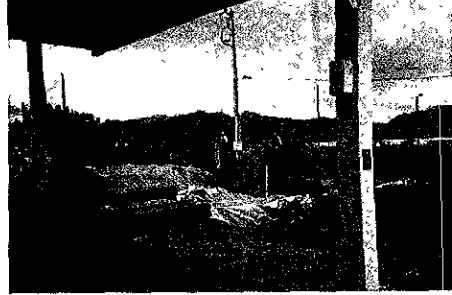
View under canopy Note metal shoring Tuesday, April 2, 2002 Sunol Tree Service; 304 Andrade Road, Sunol, California
