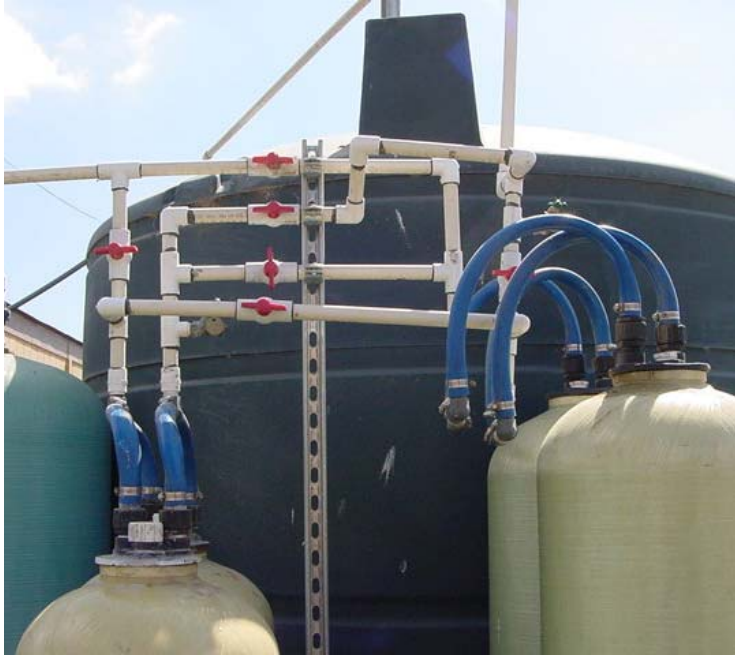
h--Bypass piping-following Carbon changeout
