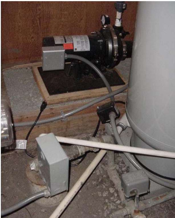
k--Repressurization Pump and Air Bladder Tank
