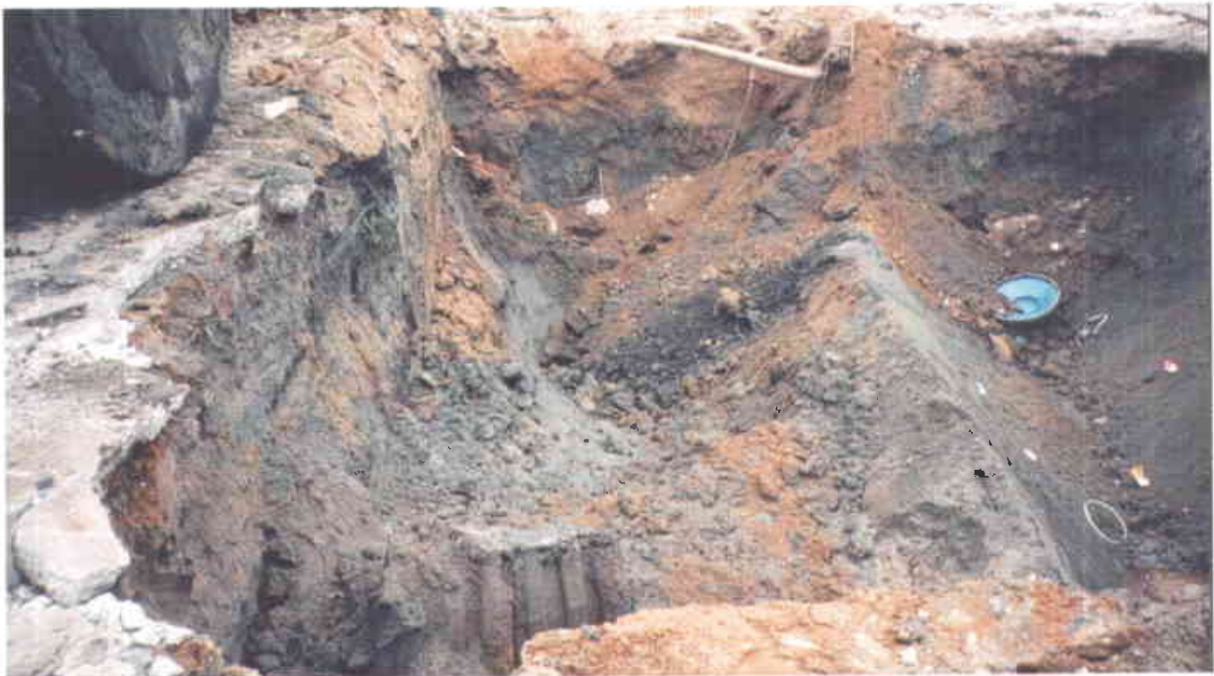
View of UST excavation cavity following removal of tanks
