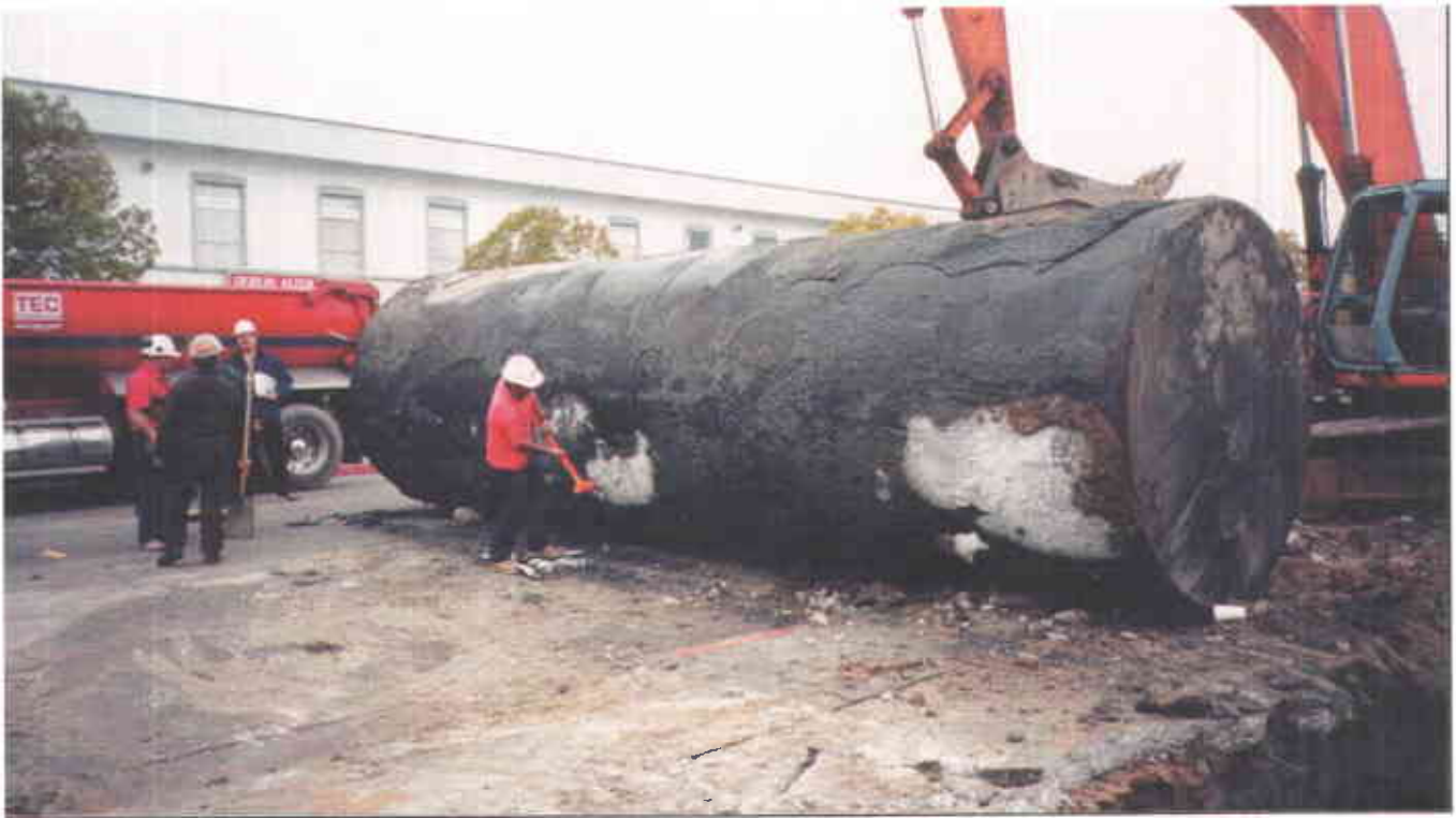
View of one of two removed USTs prior to offsite transportation of tanks.
