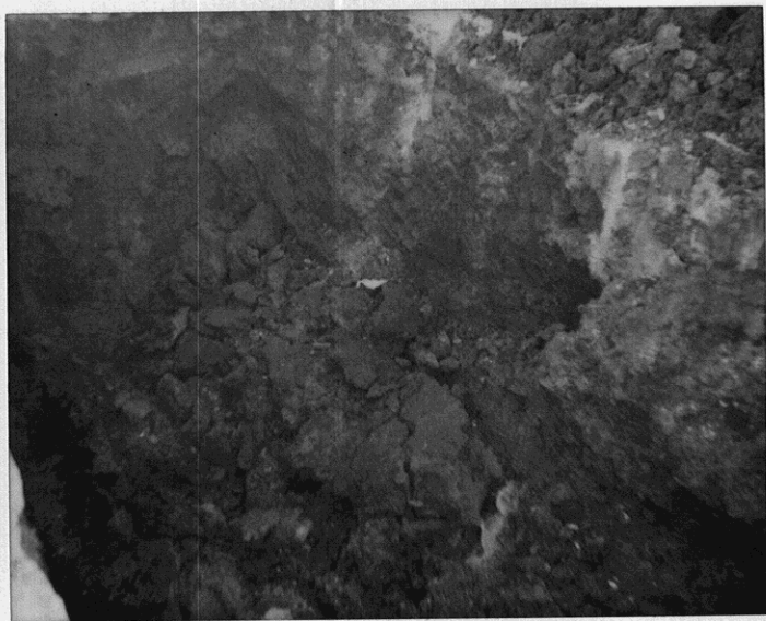
S. Side of Excavation - Tommyn's Auto Body, Meekland, Hayward 1-29-91
