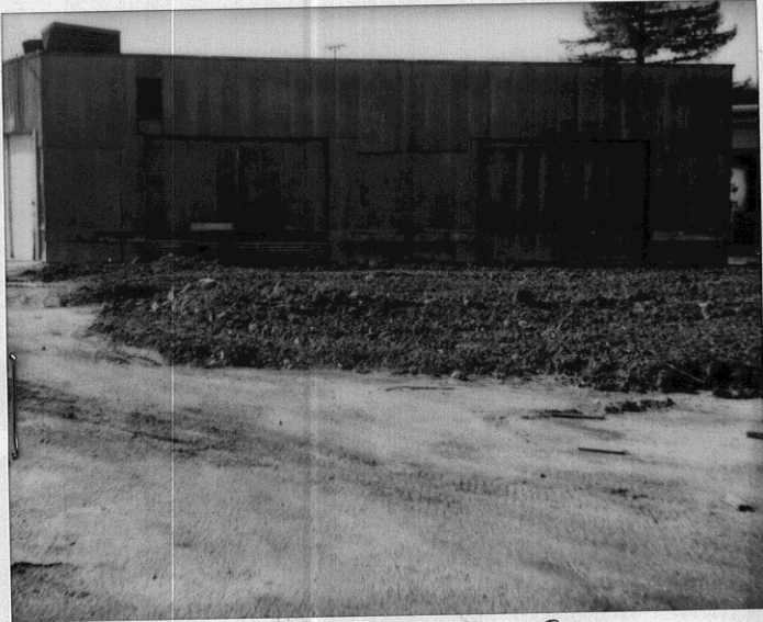
11/6/92 Brighton Ave 1259 Stockpiled Soil Albany 94706
