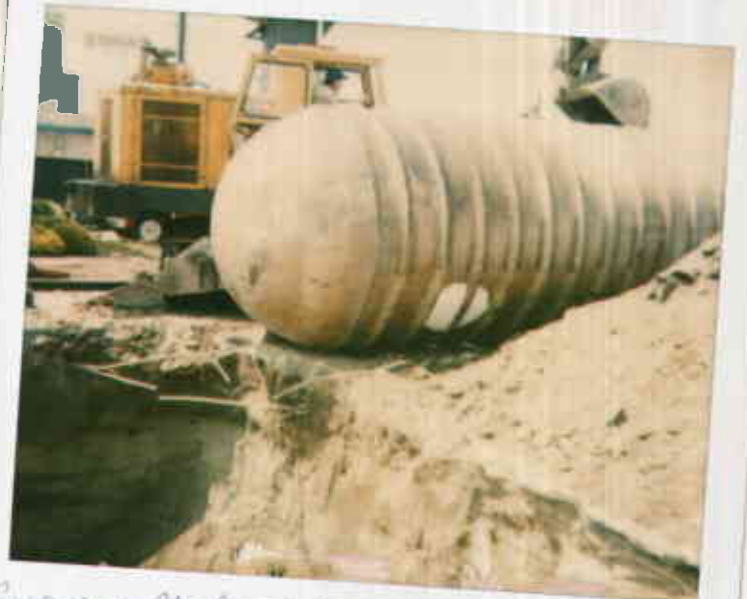
Supreme Unleaded Tank - water puddling on ground (shiny spots) Chevron, 15526 Hesperian Blvd, San Lorenzo, 5-30-91
