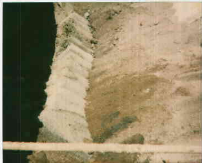
Supreme tank resting spot - dark spots appeared wet at time of removal. Chevron 15526 Hesperian Blvd, San Lorenzo. 5-30-91
