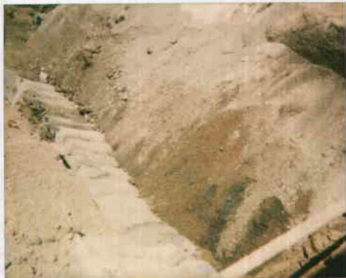
Supreme tank resting place - dark spots looked wet at time of removal. Chevron 15526 Hesperian Blvd. San Lorenzo 5-30-91
