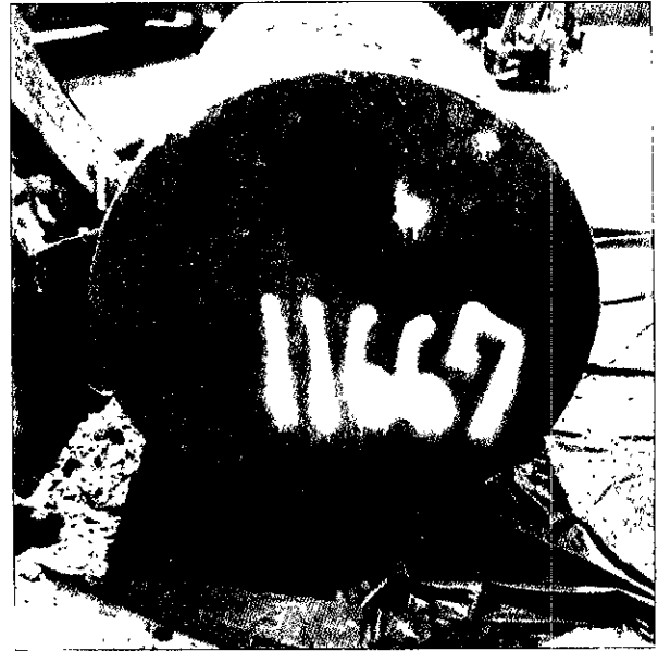
Photo 2. 550 Gallon UST After Removal.
