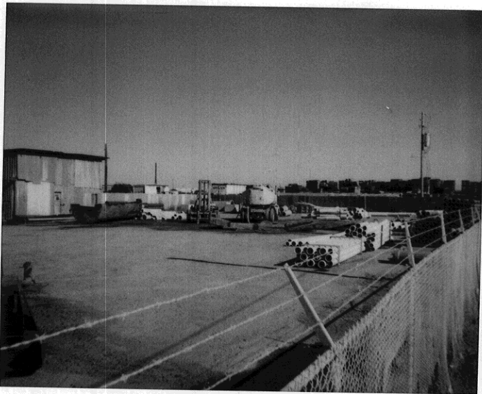
6-29-90. View from west of 3826 Depot Rd.
