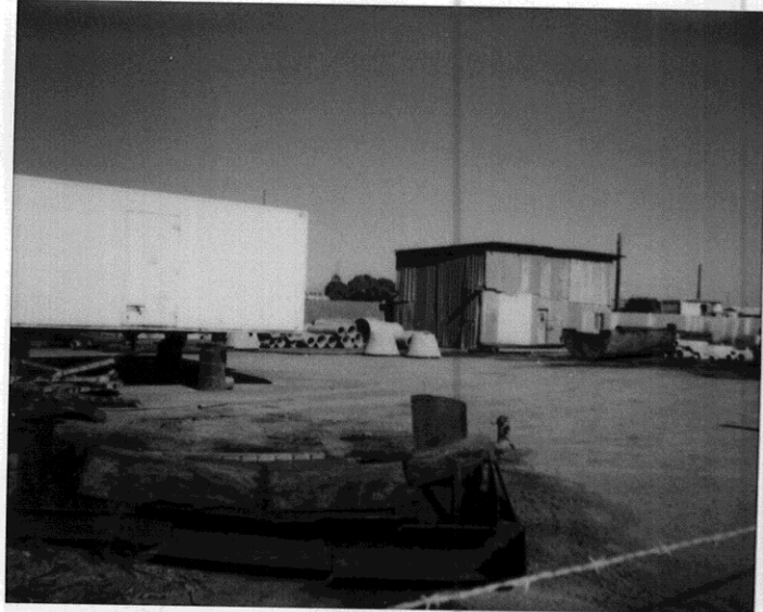
6-29-90. View from west of 3826 Depot Rd. Two tanks cut in pieces + rinsed.
