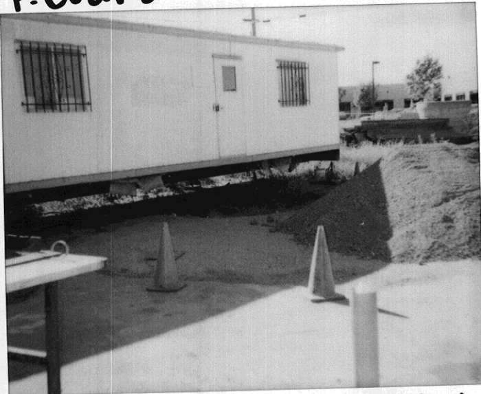
6-29-90. Excavation, refilled, at 3826 Depot Rd. Front of lot, across from office
