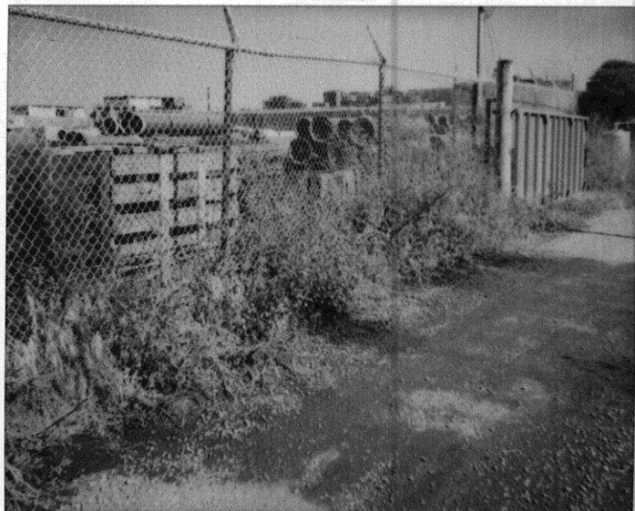
6-29-90 West of 3826 Depot Rd. Rear of lot. Mixture of water + oily liquid staining neighboring lot
