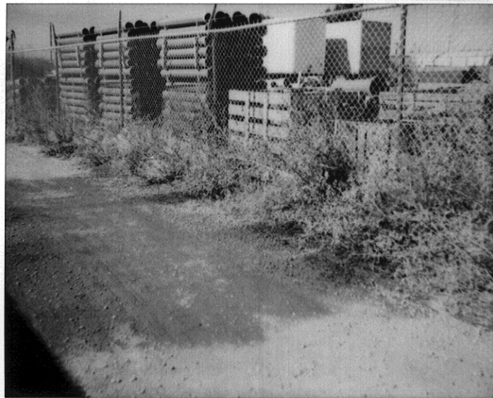
6-29-90 West of 3826 Depot Rd. Rear of lot. Mix of water + oily liquid staining neighboring lot.
