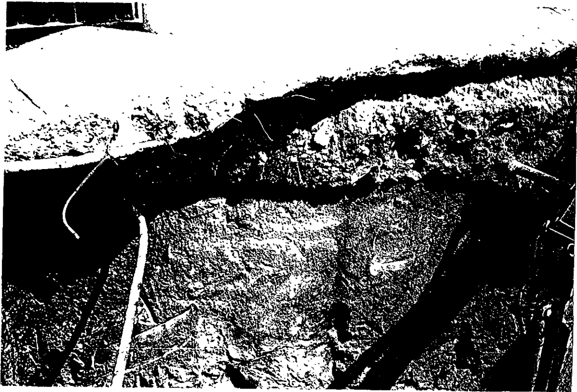
#3 East sidewall of excavation, location of two fill/return pipes
