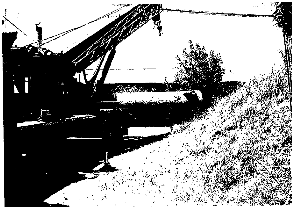
DACA-05-94-D-0012, D.O. 0005, Project No. 8808 Launcher Area, Nike Battery 31, San Leandro Removing 6,000-Gallon UST August 3, 1995, 12:35 PM, Looking South CKY, Inc. Environmental Services/Mike DeKlotz Photograph No. 2
