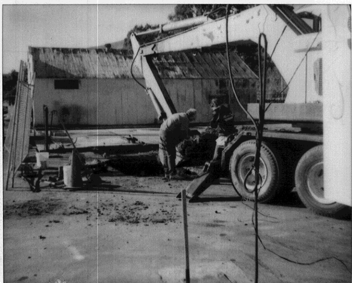
Diesel UST pit
