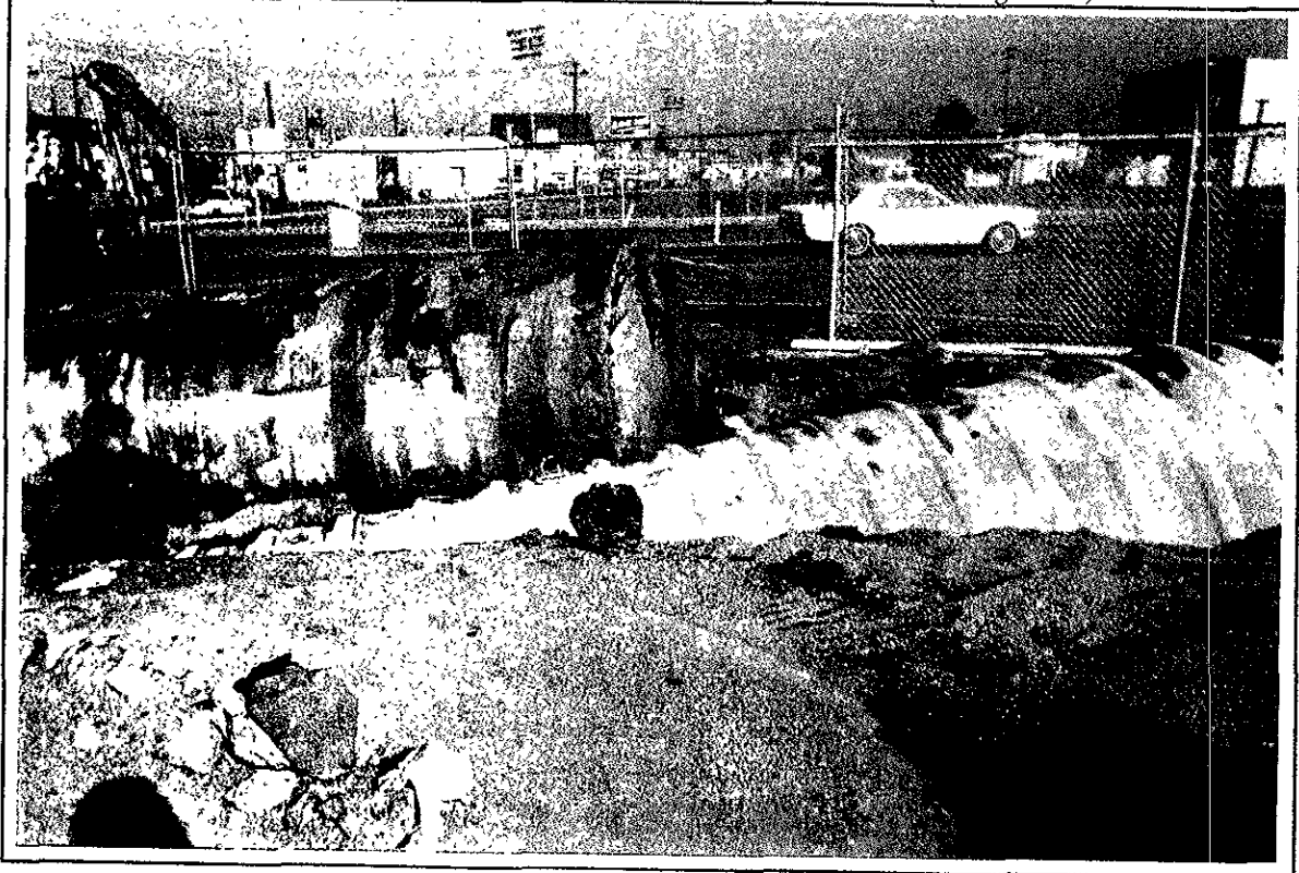
December 22, 1992: Exposed Fiberglass and Steel USTs During Excavation (facing North)
