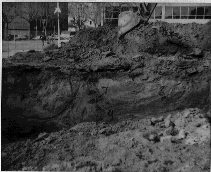
Bellevue Ave side 1/20/94 of front pit 460 Grand Ave (north side) wall
