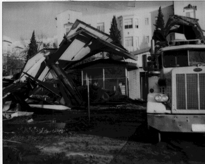
12-28-93 460 Grand Av. Oakland Station demolition!
