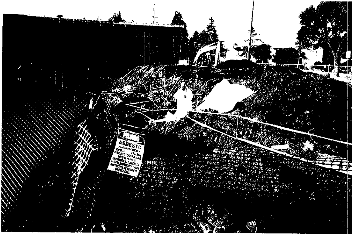
Asbestos Removal Activities: View Southwest
