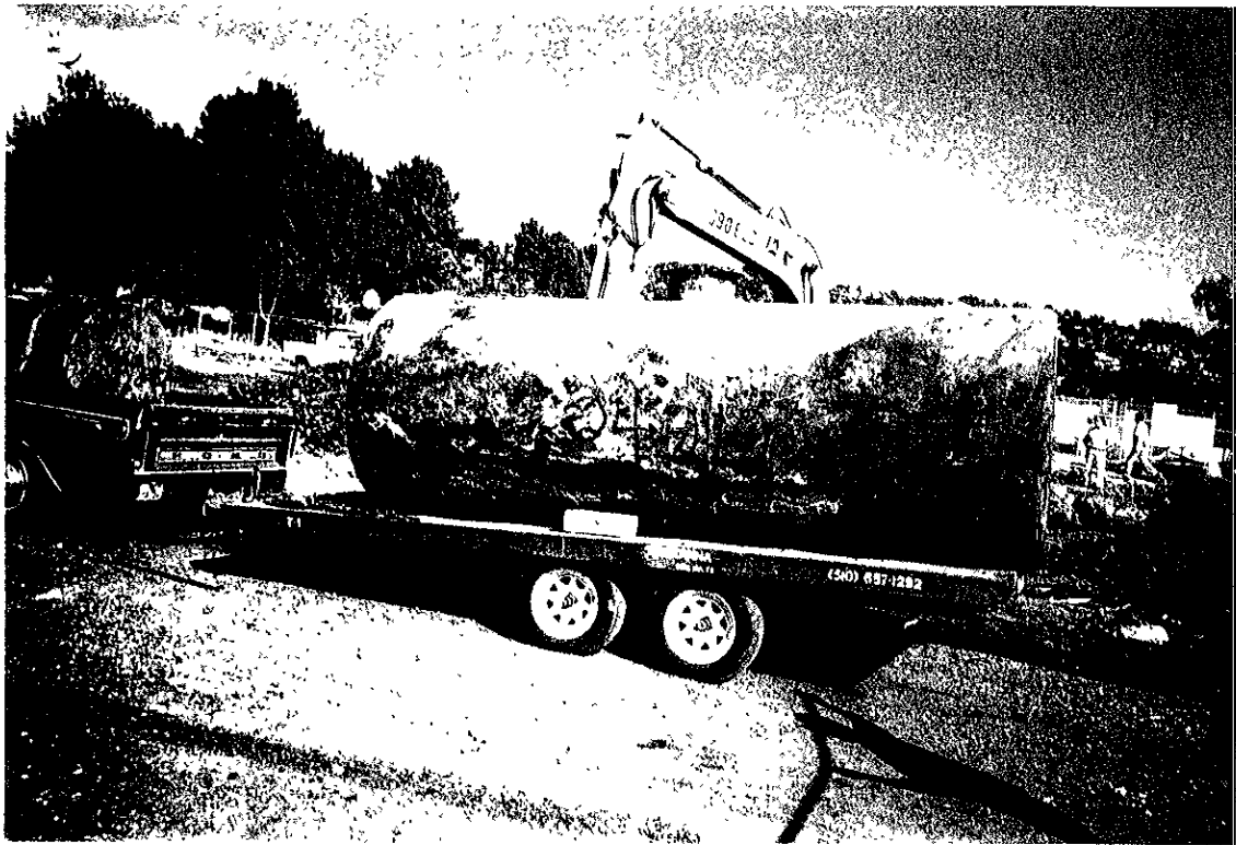
UST Loaded For Transport From the Site
