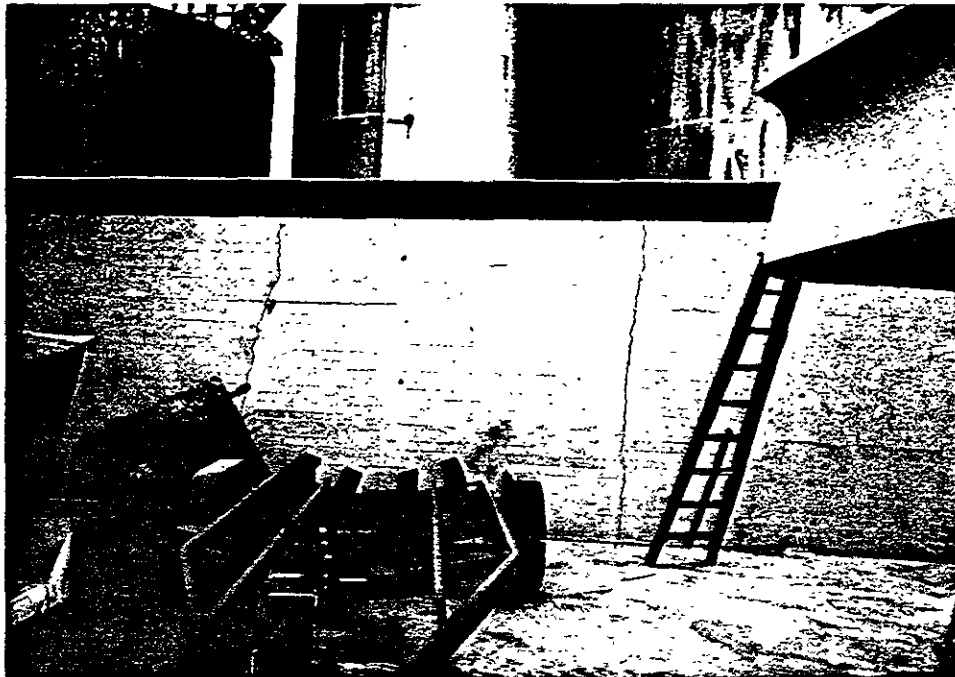
Photograph 3. Cracks in the Fuel Storage Facility Containment Wall
