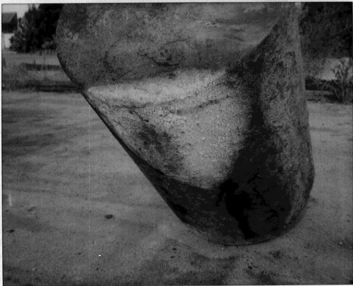
Old Santa Rita Jail Tank # 2 UST # 7 11/20/90
