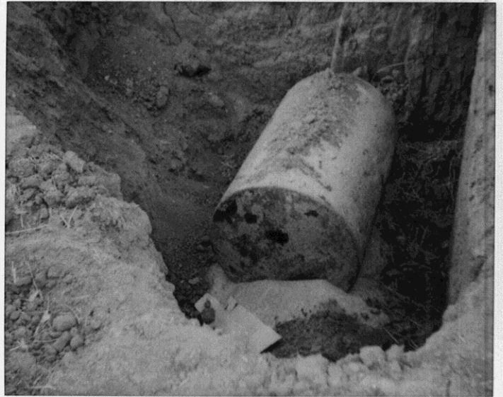
Old Santa Rita Jail Tank # 2 UST # 7 11/20/90
